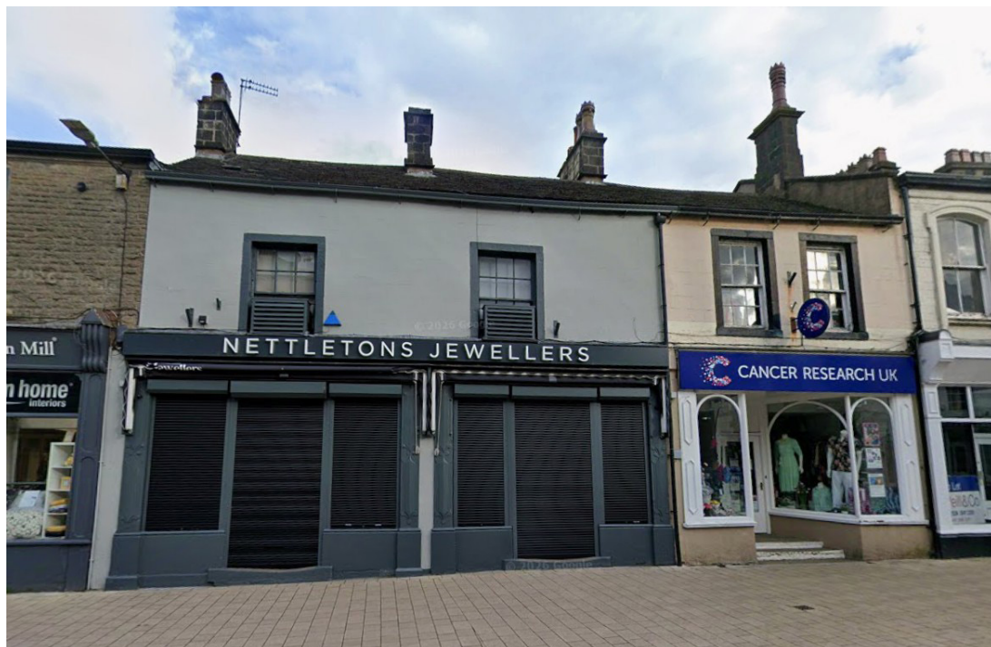
Fig 3. External photograph viewed from Castle Street (Photograph retrieved from google maps street view, 2026)
