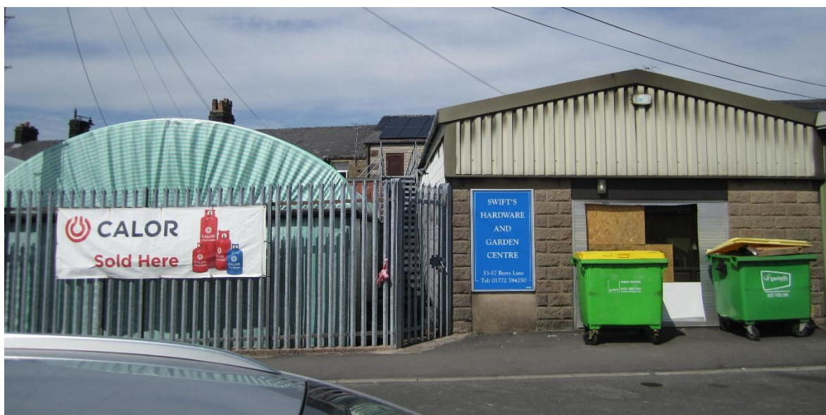
1. The application site June 2021 after the building was damaged by fire.
