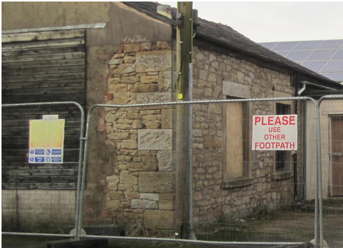
1. Detailing on the stone quoins on the corner of the building.
