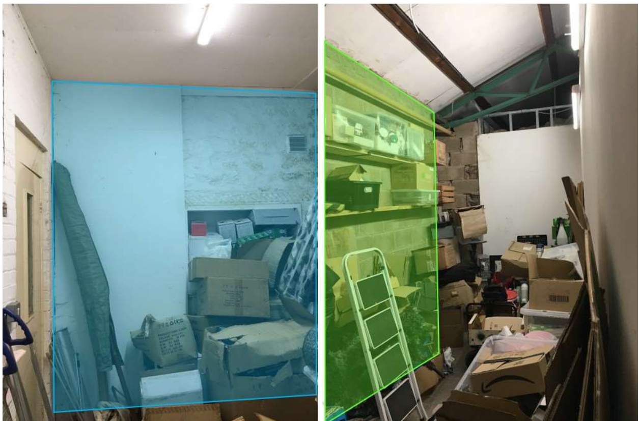
Figure 6: Photos of west party wall (highlighted blue) and north party wall (highlighted green)
