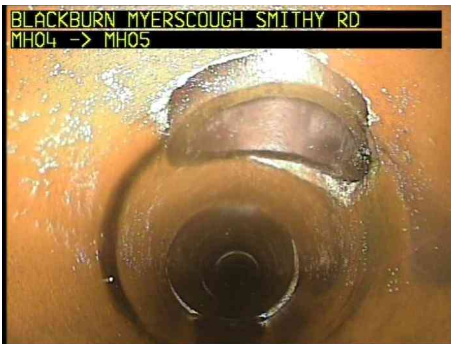
MH04X_D_13082025_1054_029.jpg, 00:00:54, 7.63 m Connection defective, connecting pipe is intruding at 12 o'clock, 100mm dia, intrusion: 5%
