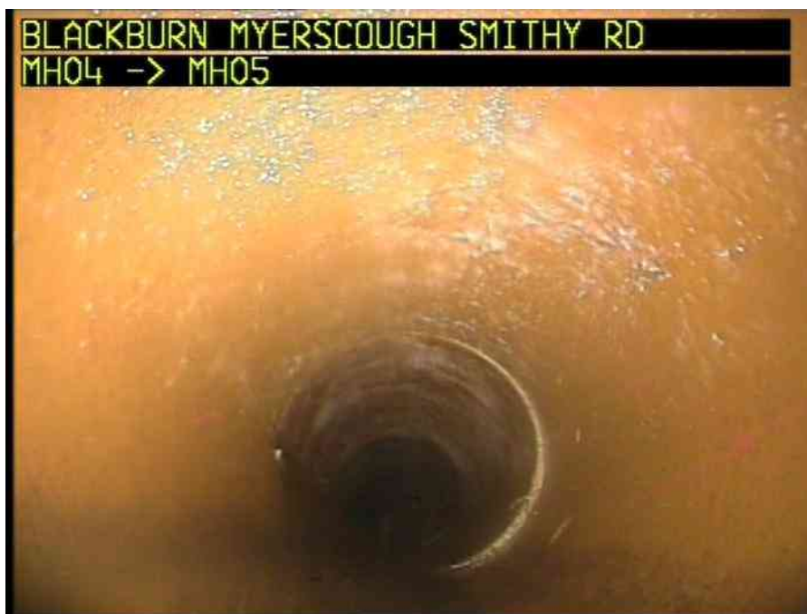
MH04X_D_13082025_1054_027.jpg, 00:00:29, 5.11 m Settled deposits, coarse, 5% cross-sectional area loss
