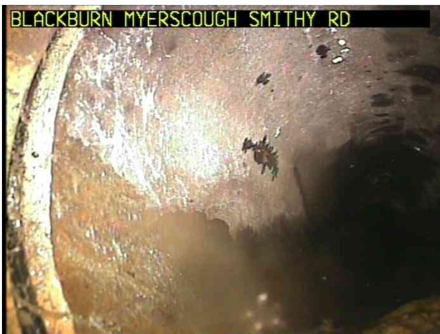
MH02X_D_13082025_1042_023.jpg, 00:00:41, 1.60 m Settled deposits, coarse, 10% cross-sectional area loss
