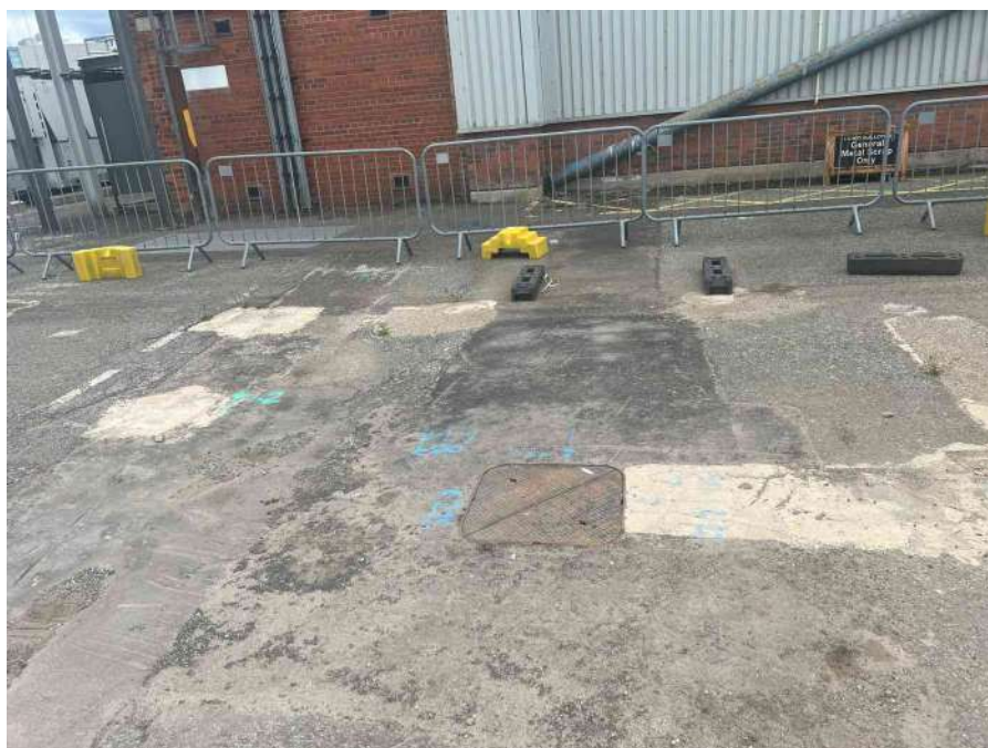
MH09X_D_14082025_1220_051.jpg, 00:00:27, 2.48 m Finish node, manhole, reference: MH08
