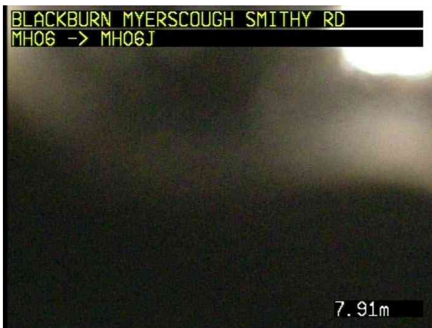
MH06X_D_13082025_1145_038.jpg, 00:00:57, 7.91 m Survey abandoned, CLEANSE REQ
