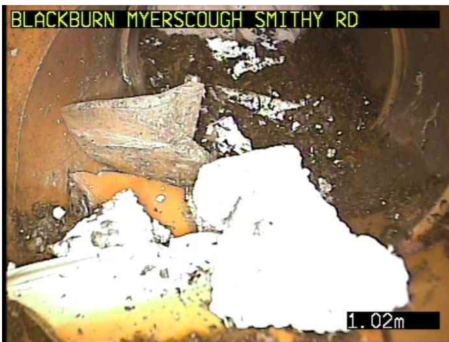
MH01AX_U_13082025_0954_008.jpg, 00:00:21, 1.02 m Settled deposits, other, 20% cross-sectional area loss, DEBRIS
