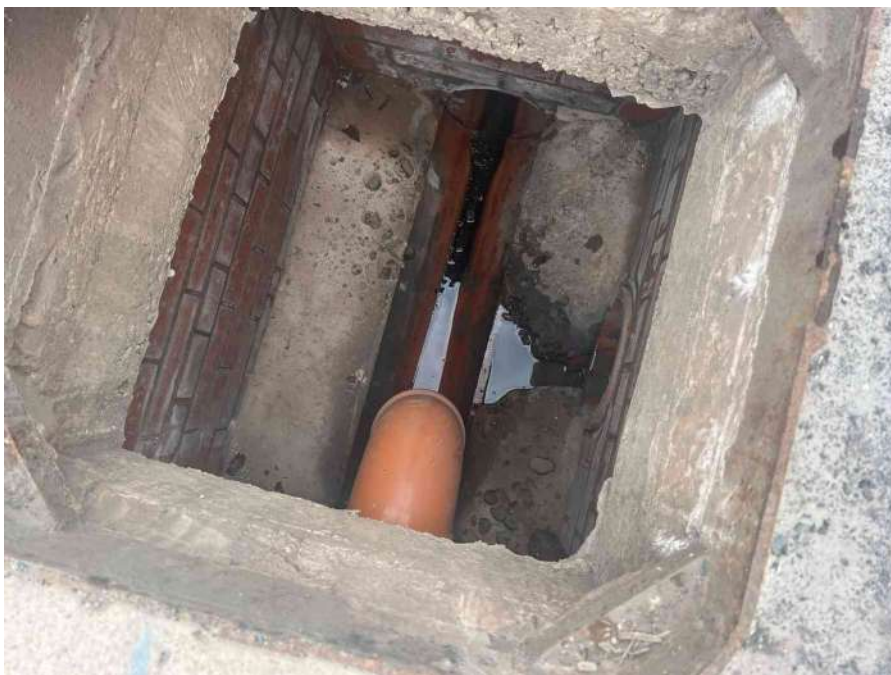
MH09X_D_14082025_1220_052.jpg, 00:00:27, 2.48 m Finish node, manhole, reference: MH08
