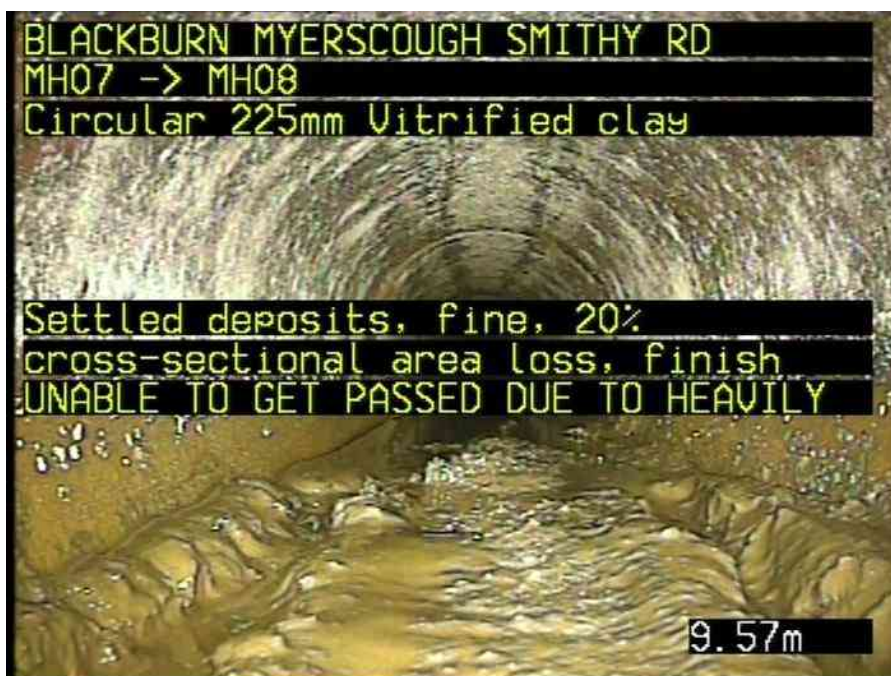
MH07X_D_14082025_1308_061.jpg, 00:01:32, 9.57 m Settled deposits, fine, 20% cross-sectional area loss, finish, UNABLE TO GET PASSED DUE TO HEAVILY SILTED
