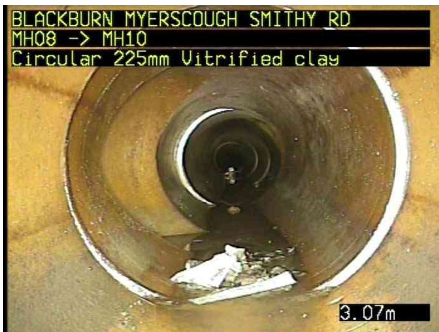
MH08X_D_14082025_1244_074.jpg, 00:00:31, 3.05 m Settled deposits, coarse, 5% cross-sectional area loss
