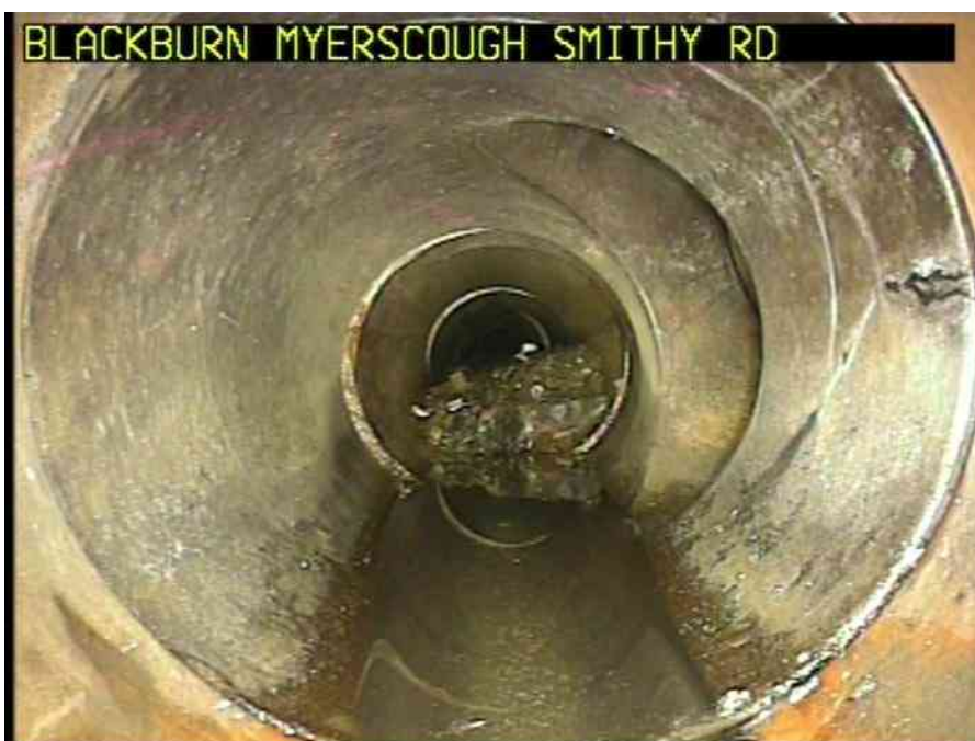
MH07X_U_14082025_1229_056.jpg, 00:00:15, 0.70 m Fracture, longitudinal at joint at 2 o'clock
