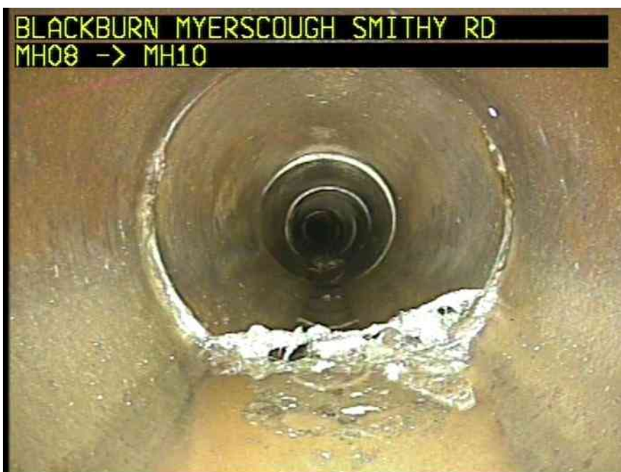
MH08X_D_14082025_1244_081.jpg, 00:06:03, 32.31 m Attached deposits, encrustation from 4 o'clock to 8 o'clock, 5% cross-sectional area loss
