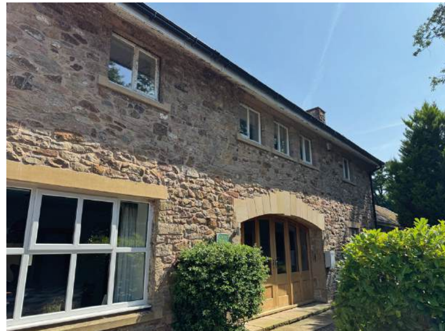
Existing stone arch and corbelled roof overhang
