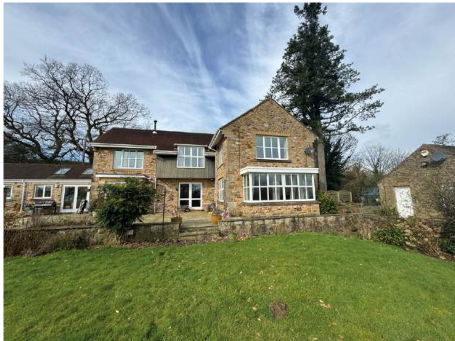
Rear elevation showing flat roof bays
