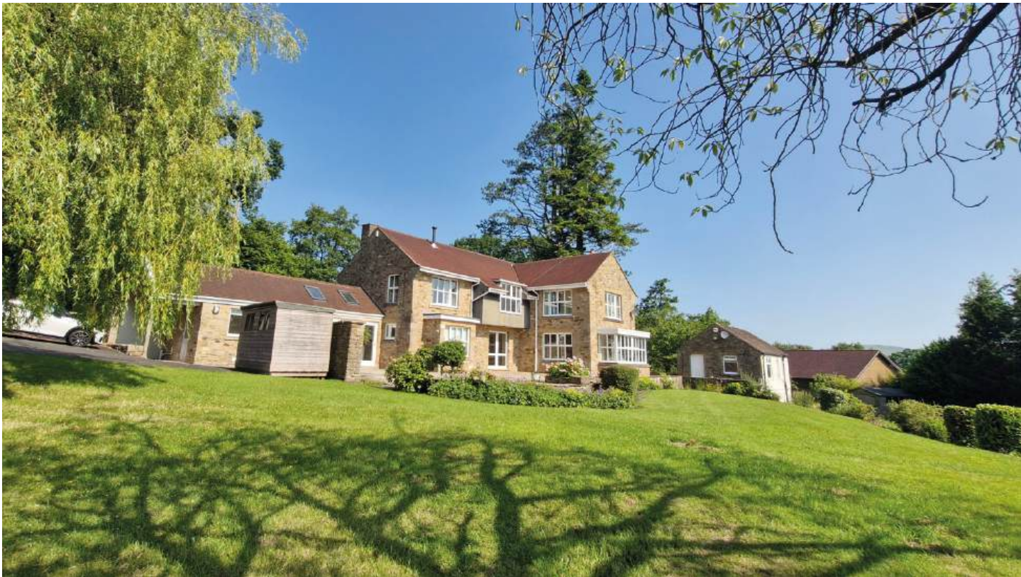
View of Existing Dwelling from South East
