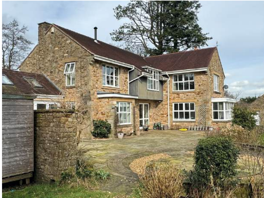
Inelegant 'flying' rear extension with upvc guttering
