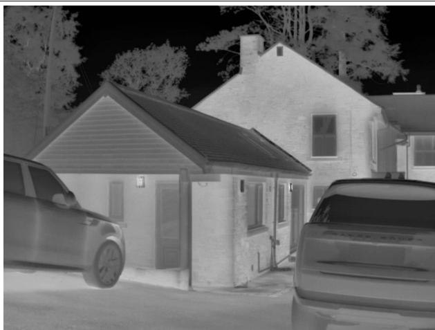
Thermal camera coverage
