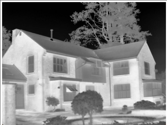
Thermal camera coverage
