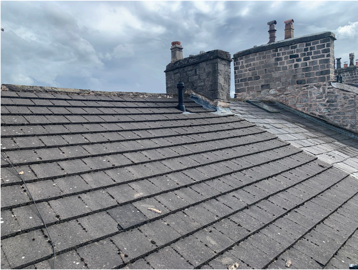
Rear roof with natural slates over no. 21 york street (5 august 2026)
