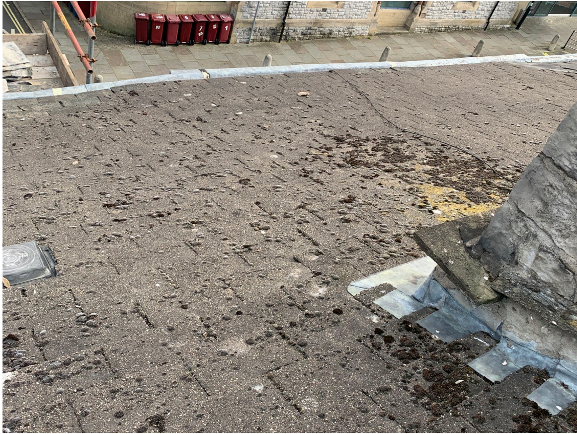
Front roof to 21 york street 5 august 2026)
