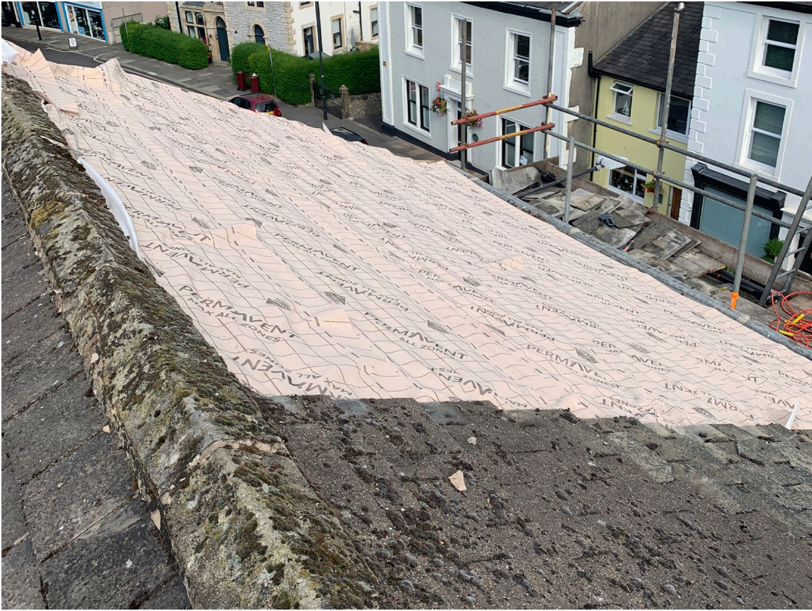
Roof stripped to half of 23 york street (5 august 2026)
