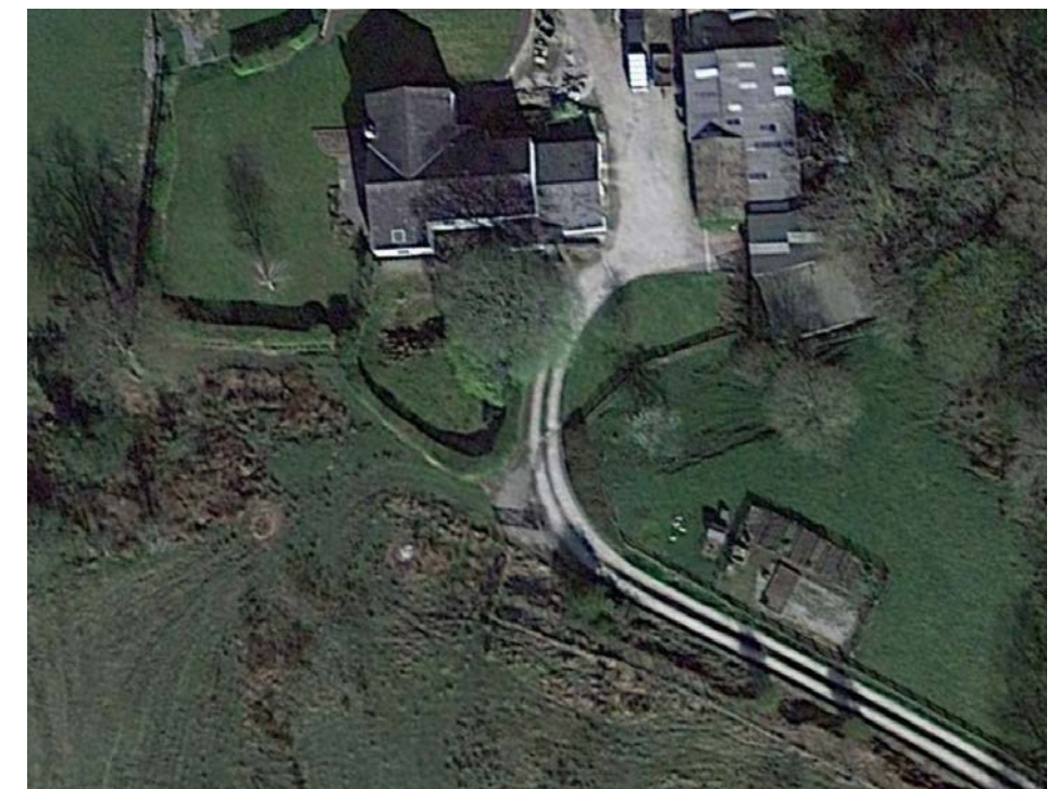
Aerial shows the existing shared access lane is natural stone with a central verge.
