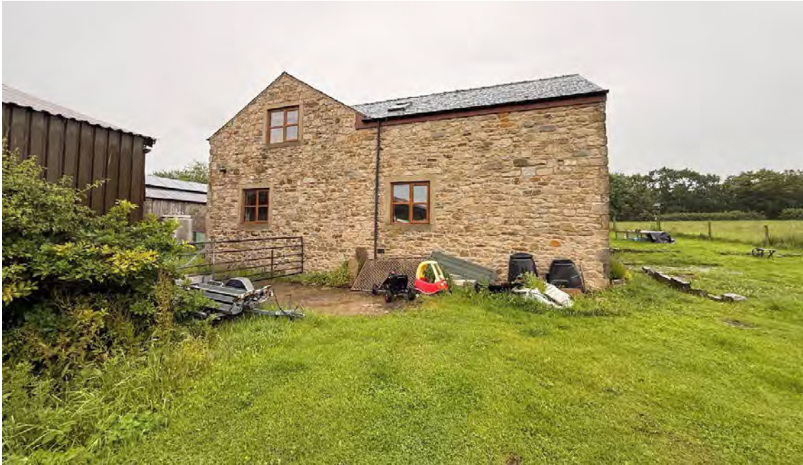
As built photographs dated 2026
