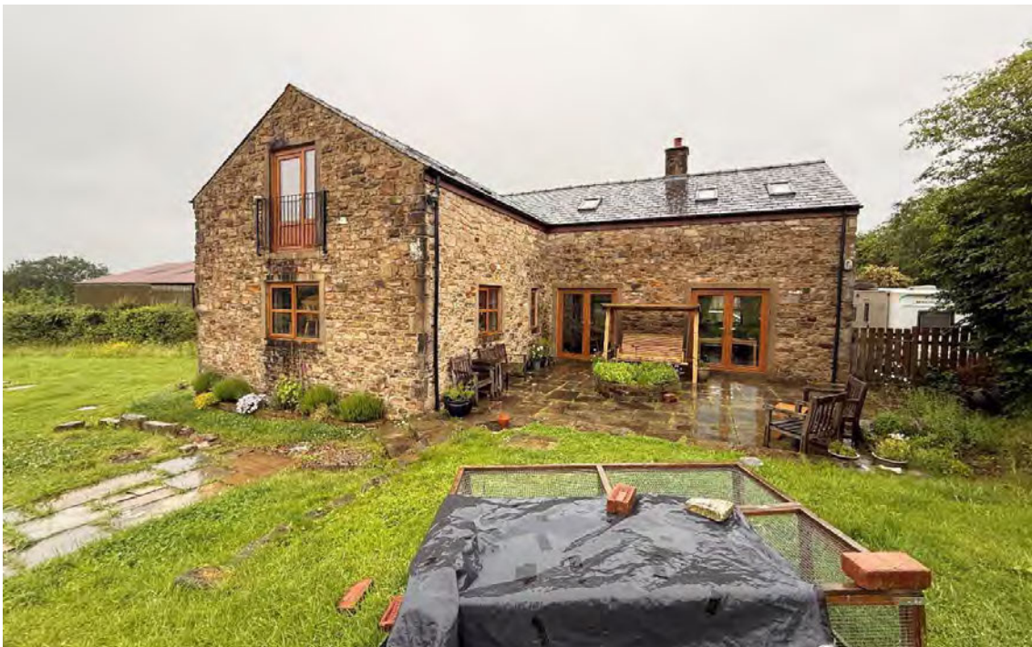
As built photographs dated 2026
