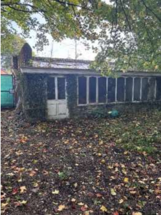
Photograph 13: Building 1 with negligible bat roost potential.
