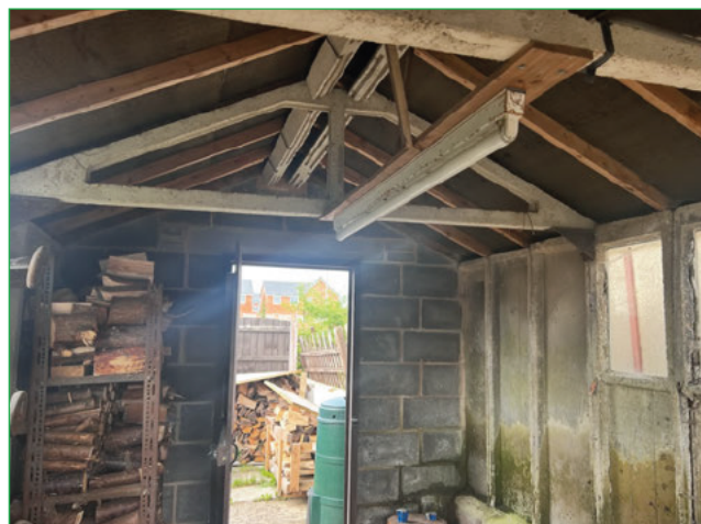
Showing the interior of Garage A
