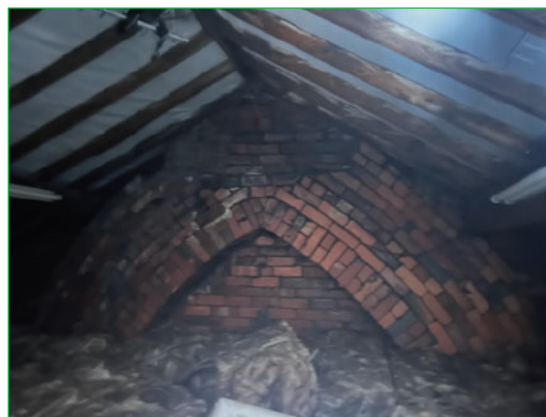
The large loft void, well-sealed from the exterior. No bats or droppings were found
