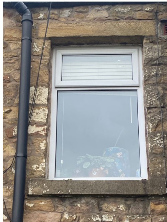
First floor rear elevation window
