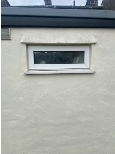
Ground floor rear elevation Shower room window.
