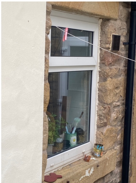
Ground floor rear elevation kitchen window.
