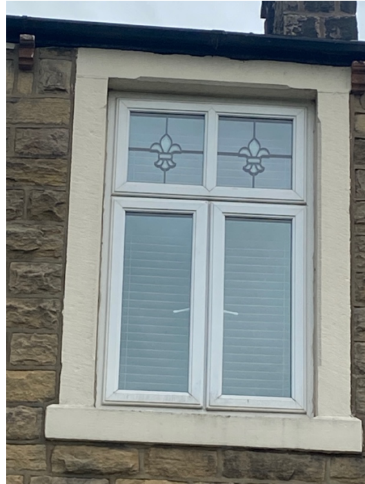
First floor front elevation window
