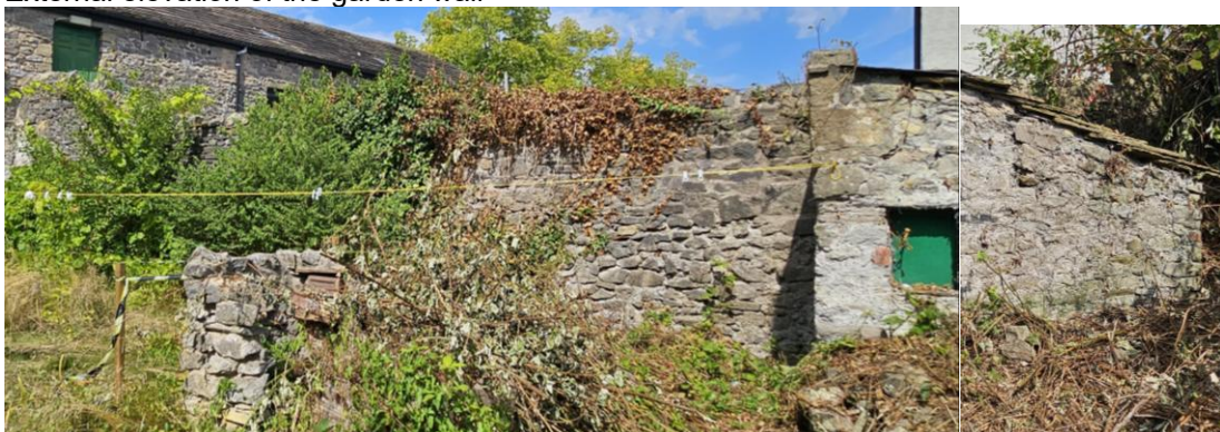
Internal view of the wall and small garden store. The garden wall is immediately adjacent to the store and forms its northeast wall.
