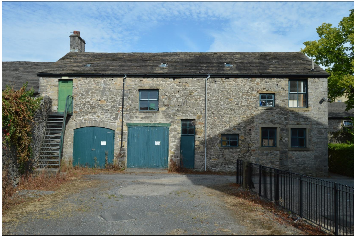
PL09: View of The Old Stables from the southeast.
