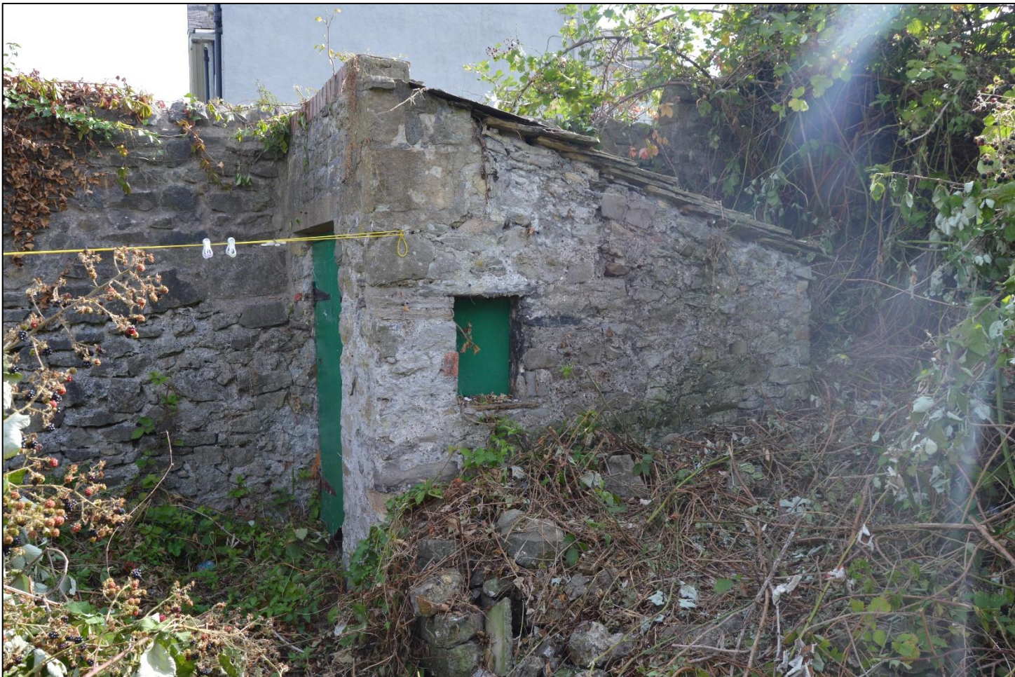
PL06: View of the stone storage shed adjoining the southwest side of the wall at its southeast end.
