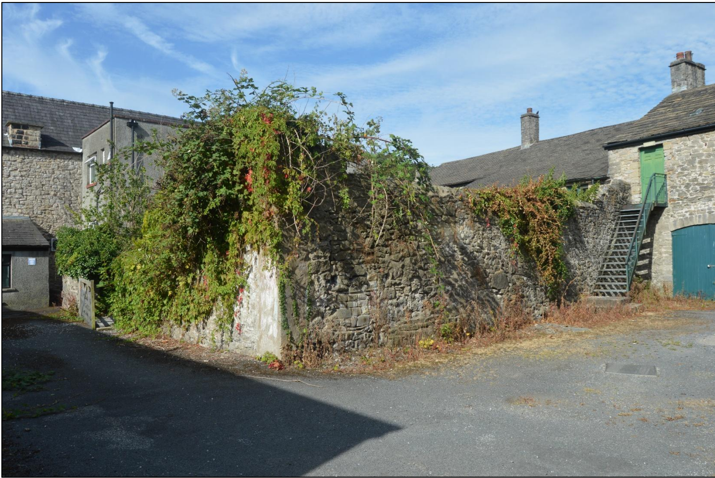
PL02: View of the boundary wall from the east.
