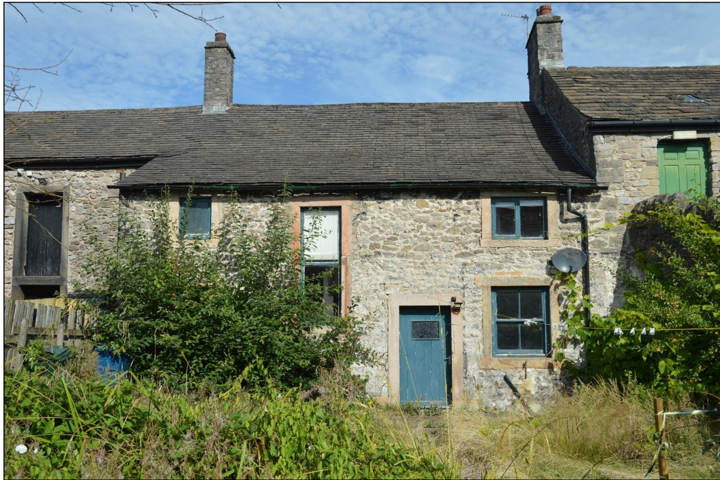
PL11: View of No.41 Lowergate (Dower House) from the southeast.
