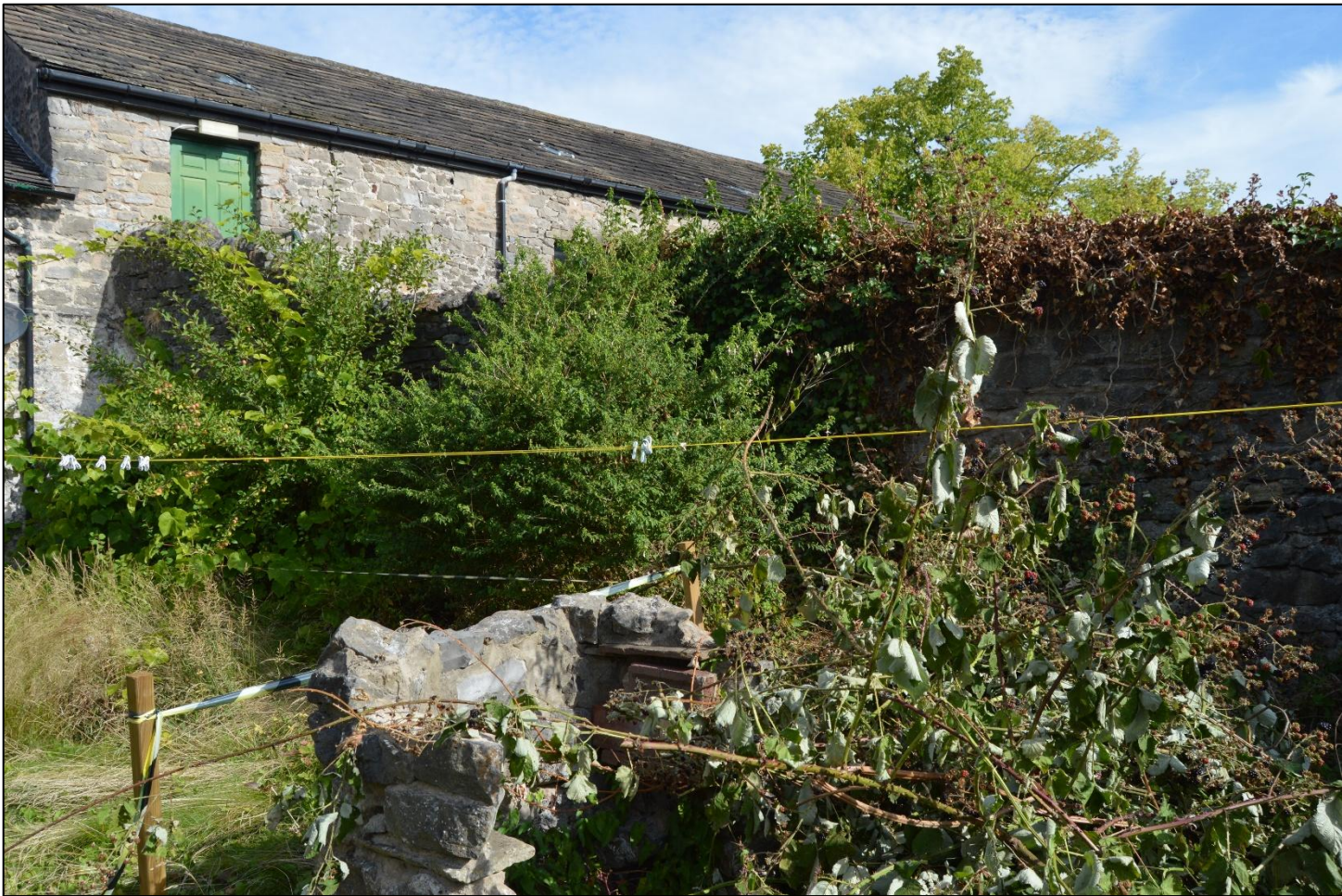
PL04: View of the boundary wall from the south.
