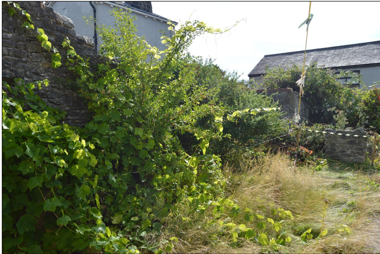
PL03: View of the boundary wall from the northwest.
