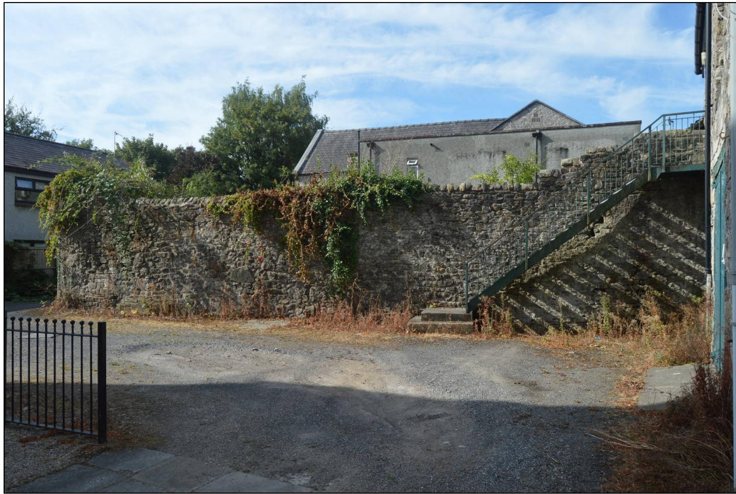
PL01: View of the boundary wall from the north-east.
