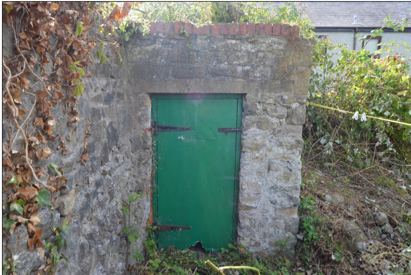
PL05: View of the stone storage shed adjoining the southwest side of the wall at its southeast end.
