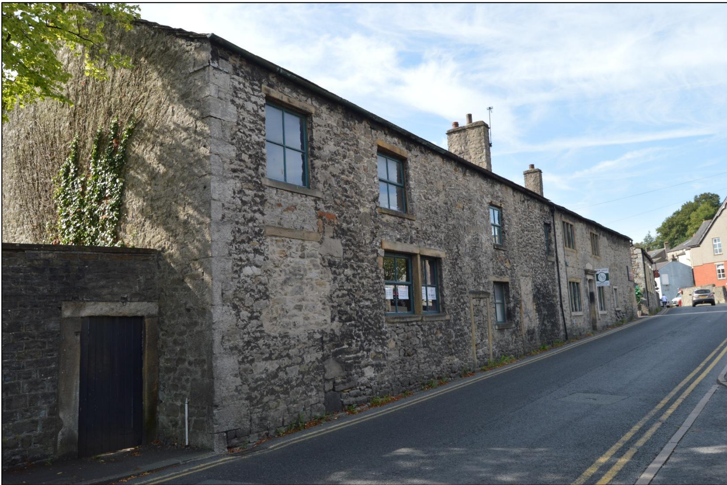
PL12: View of The Old Stables and 41 Lowergate (Dower House) from the east.
