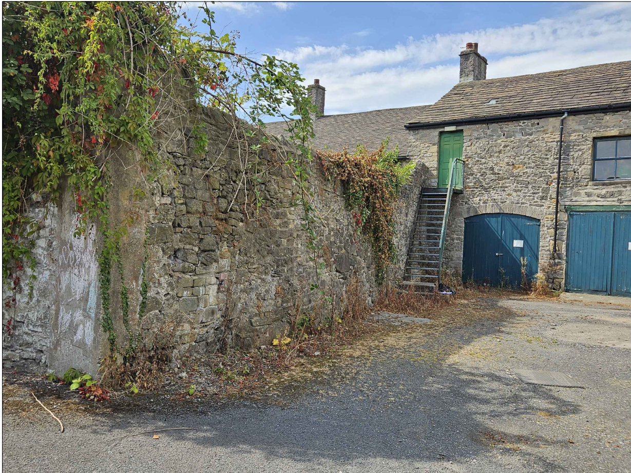
EXISTING WALL AND STAIR
