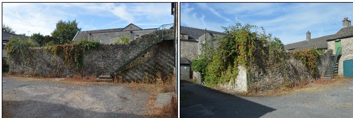
PL01: Views of the wall from the north east yard area.
