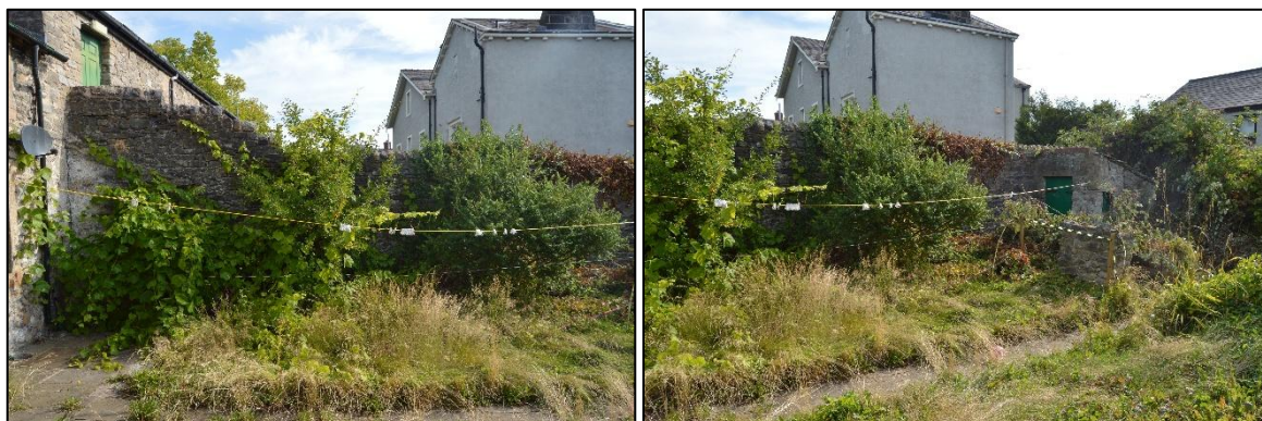
PL02: Views of the wall from the south west within the garden to No 41 Lowergate.
