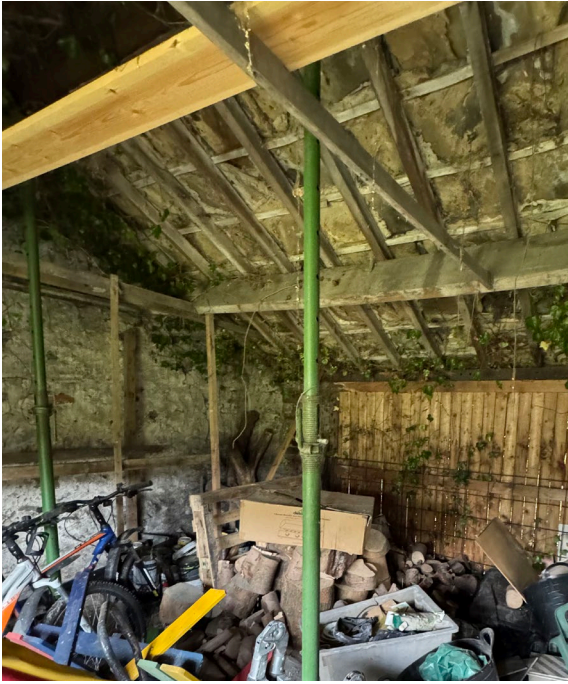
Internal view showing temporary supports
