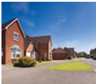
Estate & Access Roads
