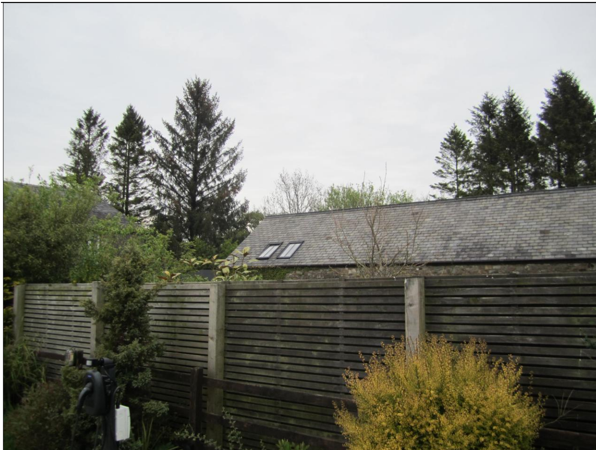
2 Rooflights in the south west elevation of the garage belonging to The Old Dairy.
