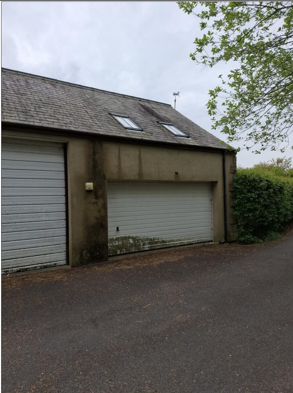
1 Rooflights in the north east elevation of the garage belonging to The Old Dairy.
