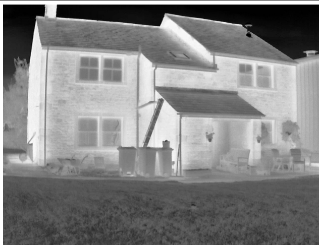
Thermal Camera Coverage
