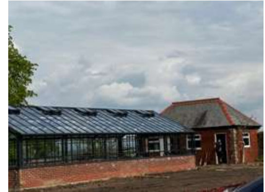
Buildings B1 and B2
