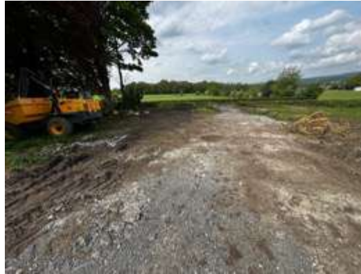
Recent site clearance
