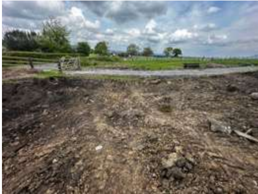
Recent site clearance
