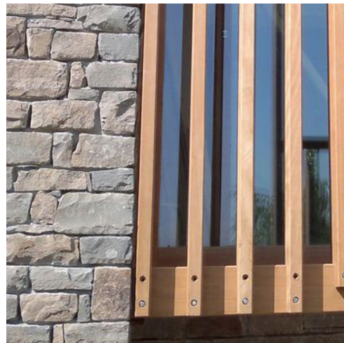
Hit & Miss Cladding Green oak slats fixed between oak frame
