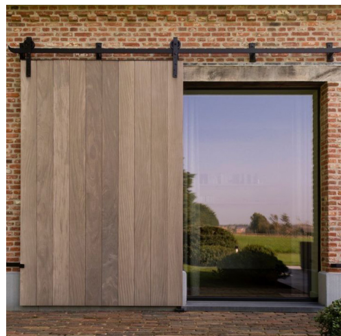
Sliding shutters Green oak shutters face fixed to stone walls in front of glazing
