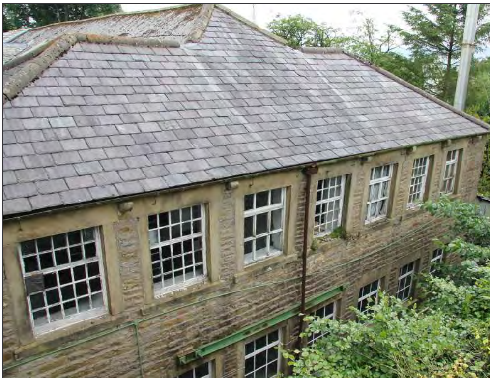
Plate 10: External west elevation of the west wing
