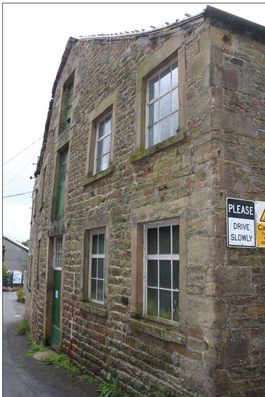
Plate 9: The eastern extension along Malt Kiln Brow
