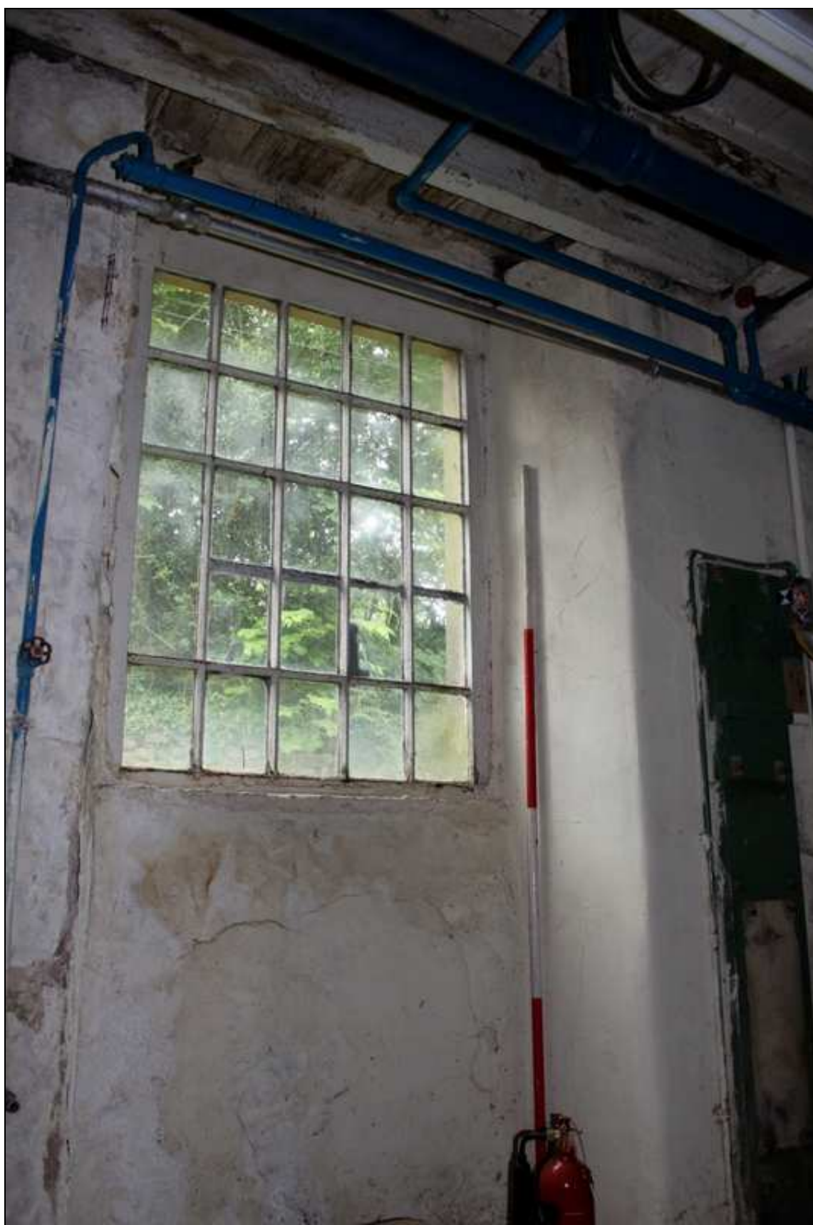
Plate 55: 25-light window in north wall, first floor
