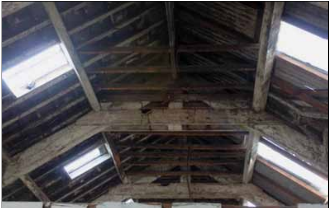
Plate 83: Remodelled king post trusses
