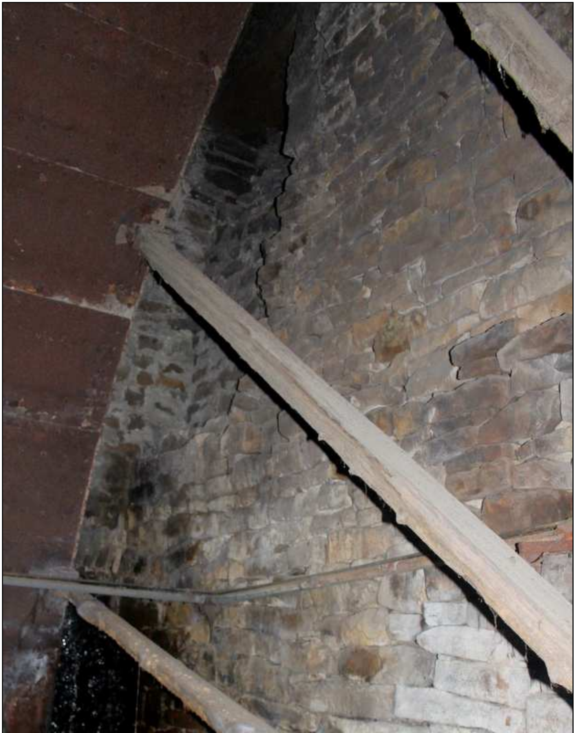
Plate 72: East wall of wheel house with quoin return of probable doorway at to
