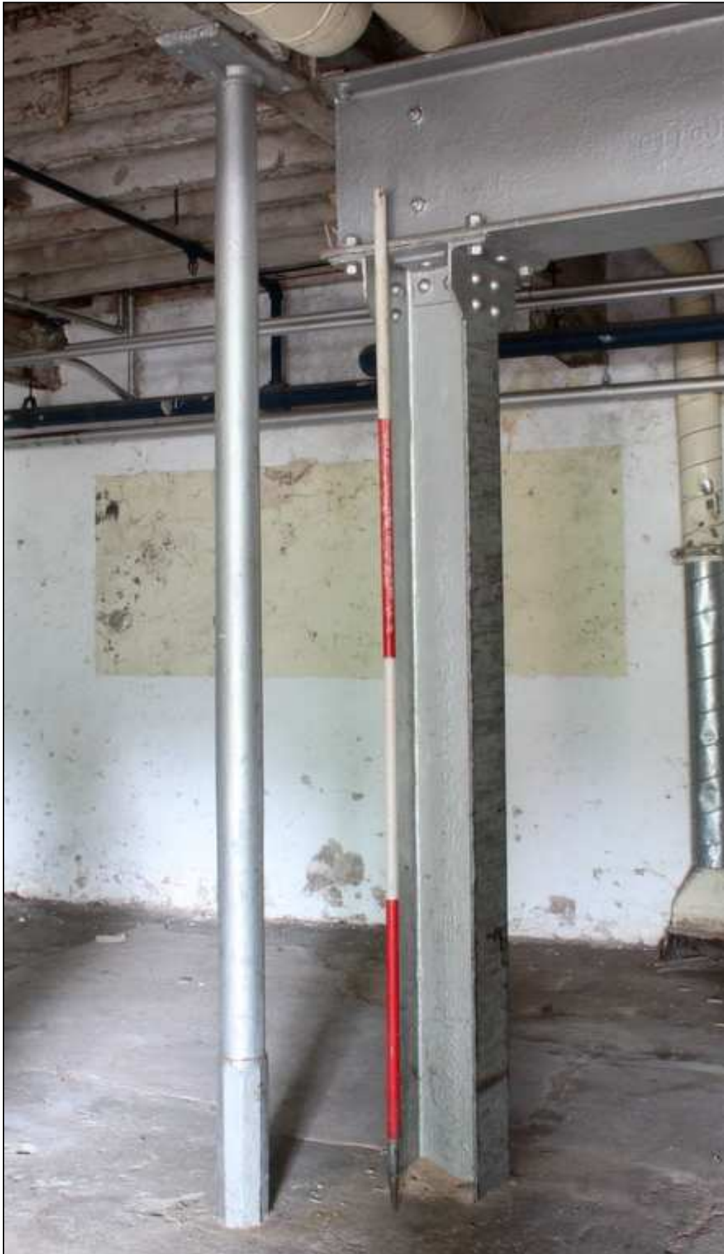
Plate 29: Detail of octagonal-section column foot
