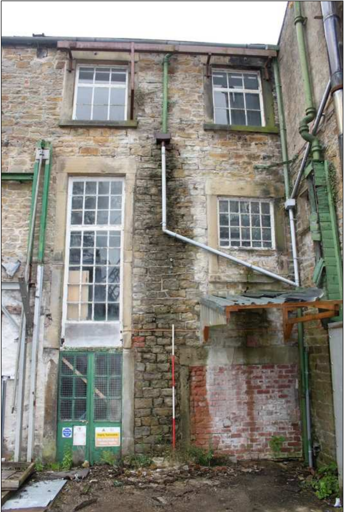
Plate 8: Façade of engine and wheel houses
