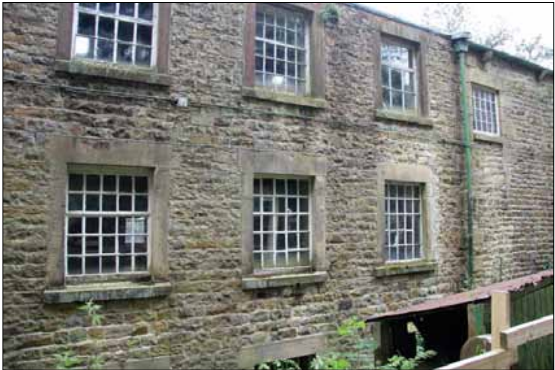
Plate 14: External elevation of repositioned north wall of main mill
