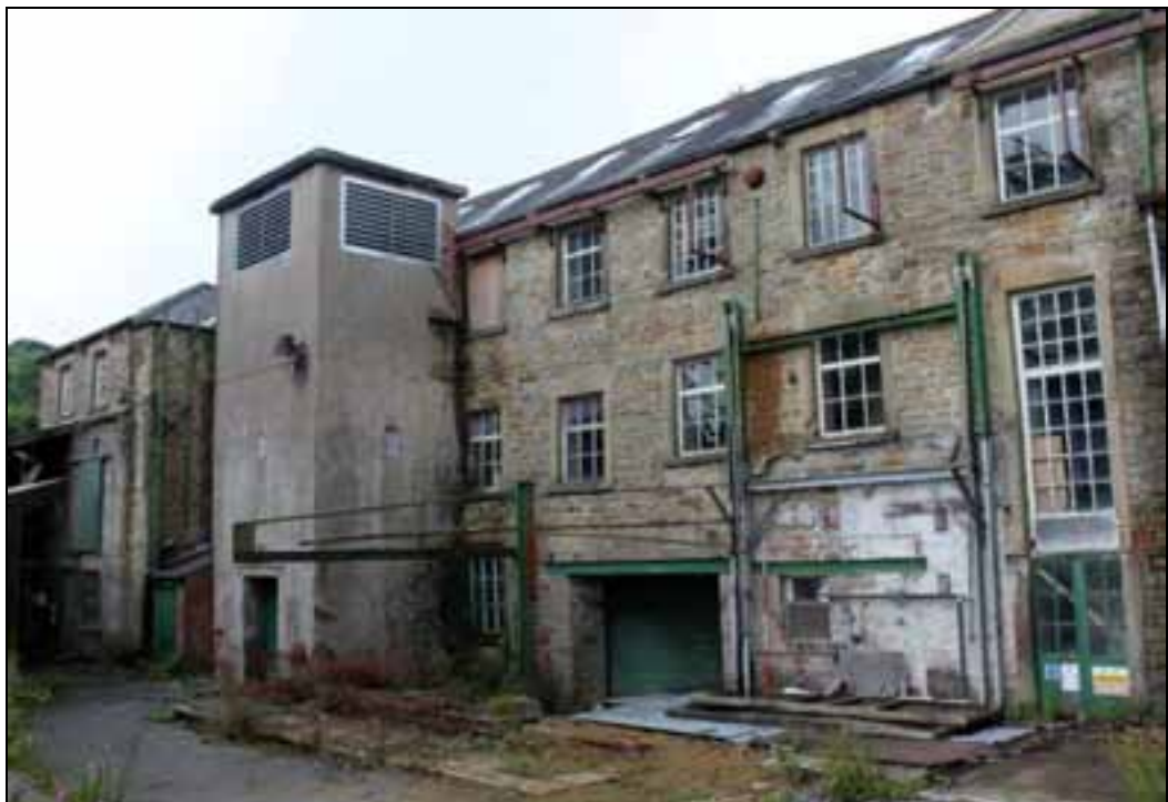
Plate 4: The south-facing elevation of Kirk Mill
