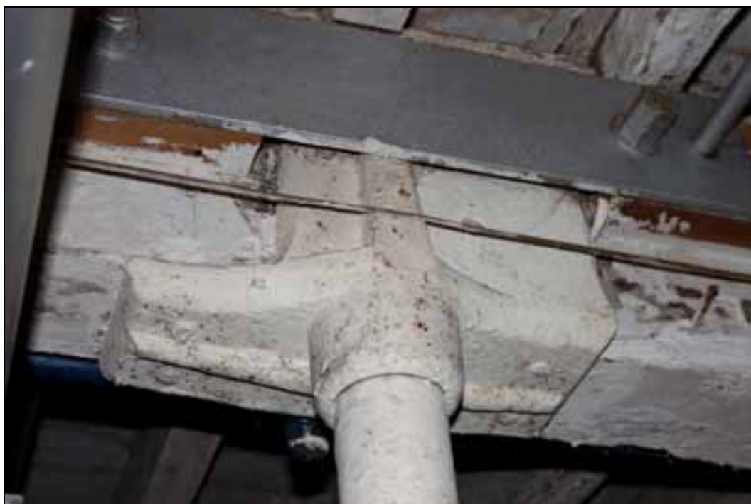
Plate 53: L-section column head plate
