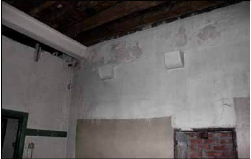
Plate 76: Sandstone corbels in south external wall of original eastern extension
