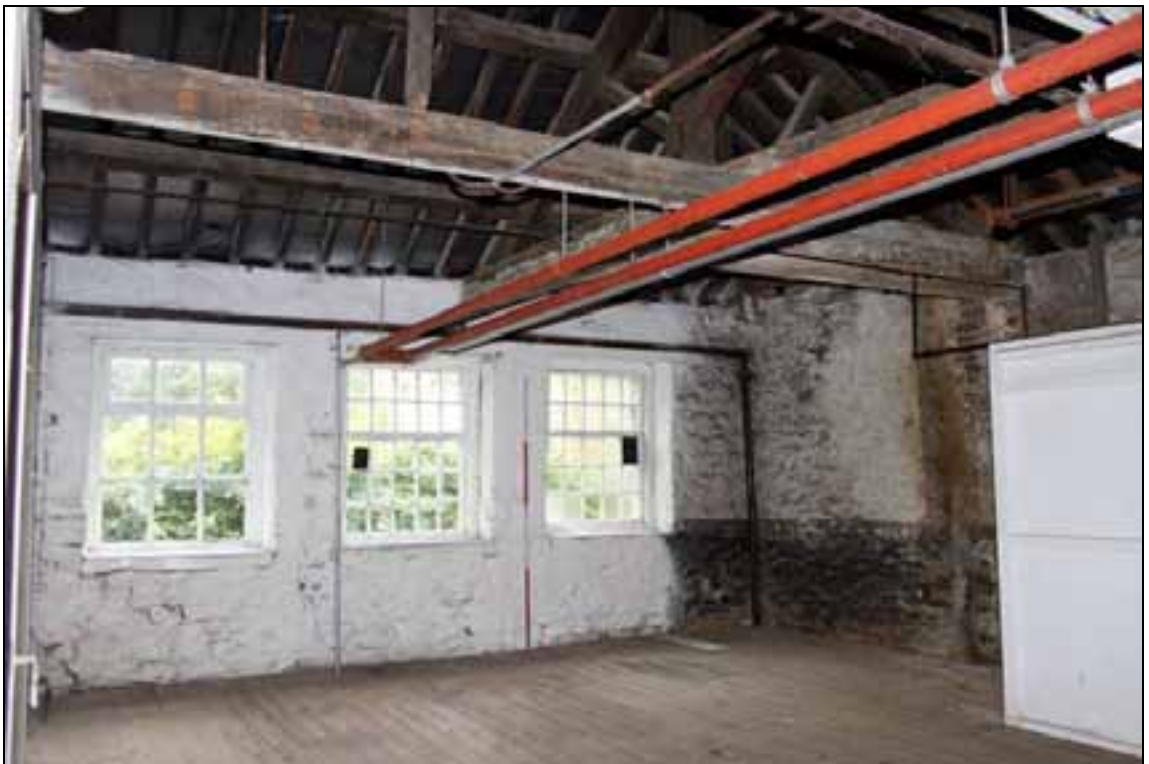
Plate 7: General view across the west wing of the second floor
