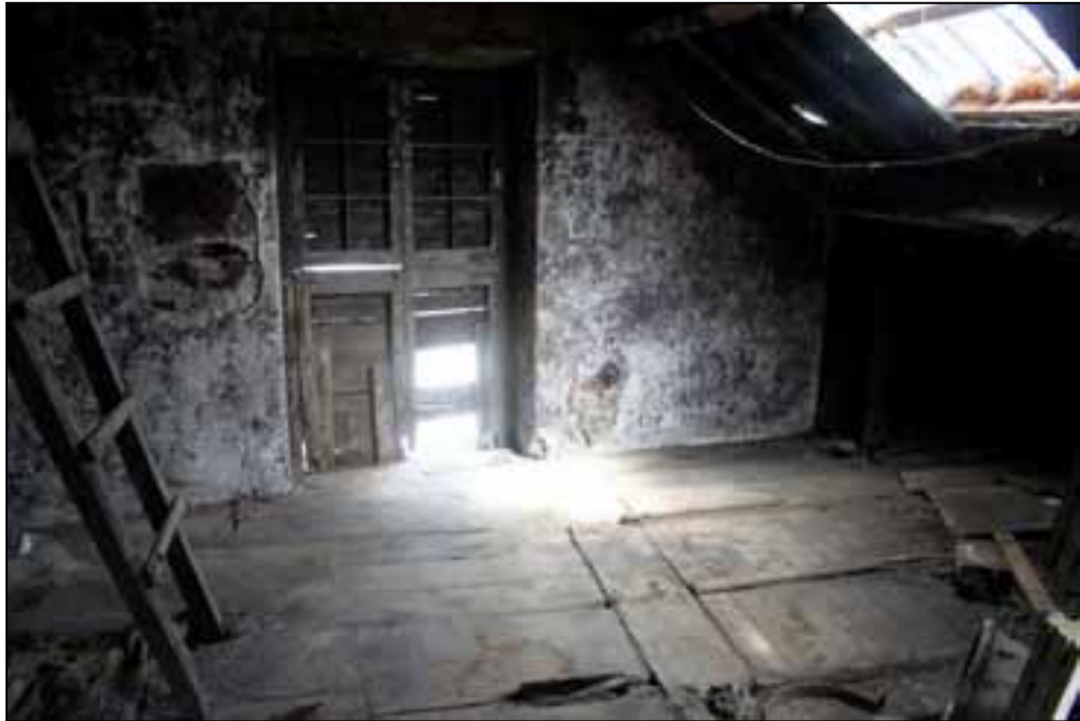
Plate 97: Loading door and associated trapdoor above east extension
