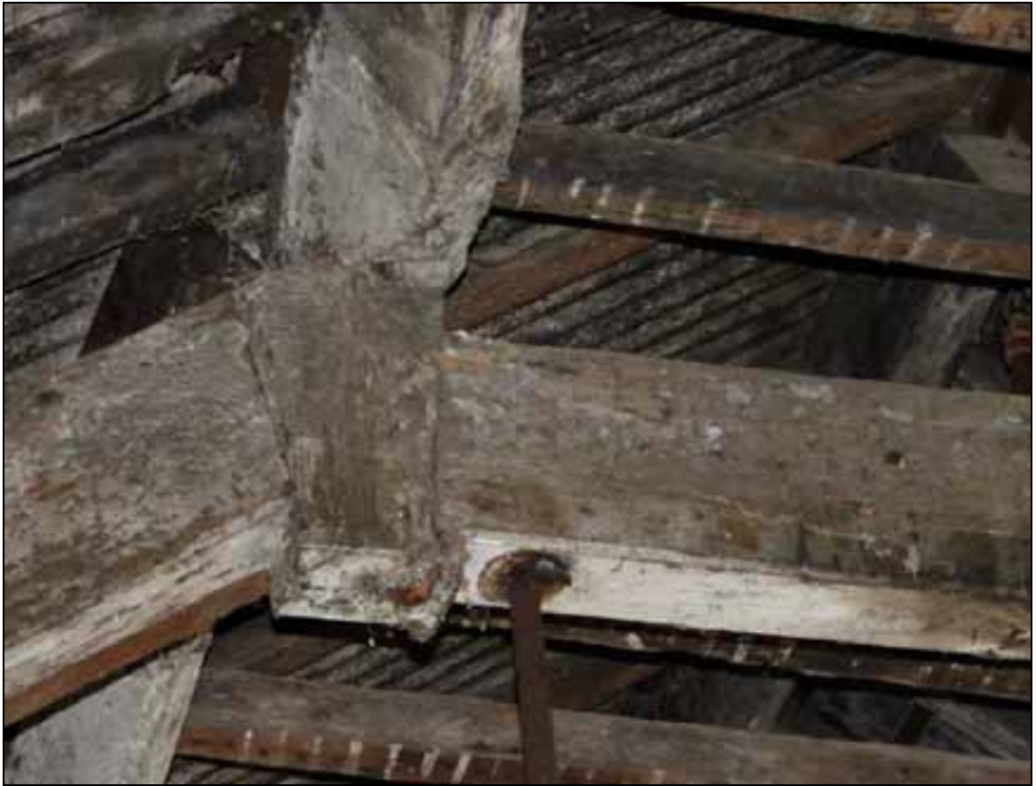
Plate 88: Jowled head of queen post, carrying side purlin, with adjacent replacement rod
