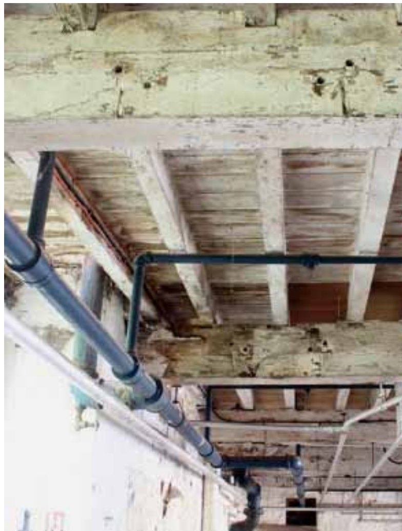
Plate 40: Bolt holes and scars for northern line shaft, with end bearing in background
