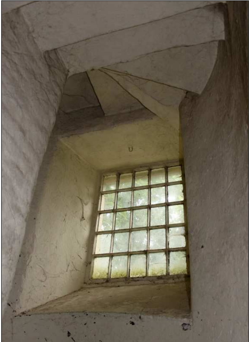
Plate 59: Stair-light window with fireproof spiral stair above
