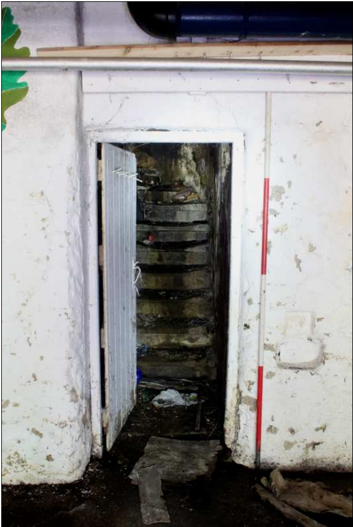
Plate 33: Base of stair tower with spiral staircase
