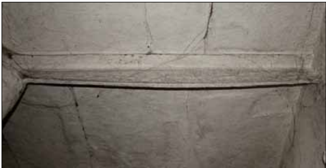
Plate 61: Fish-bellied T-section beam carrying stair tower landing
