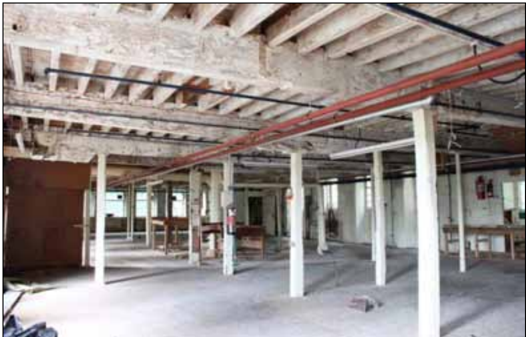
Plate 47: General view across the first floor, looking north-west
