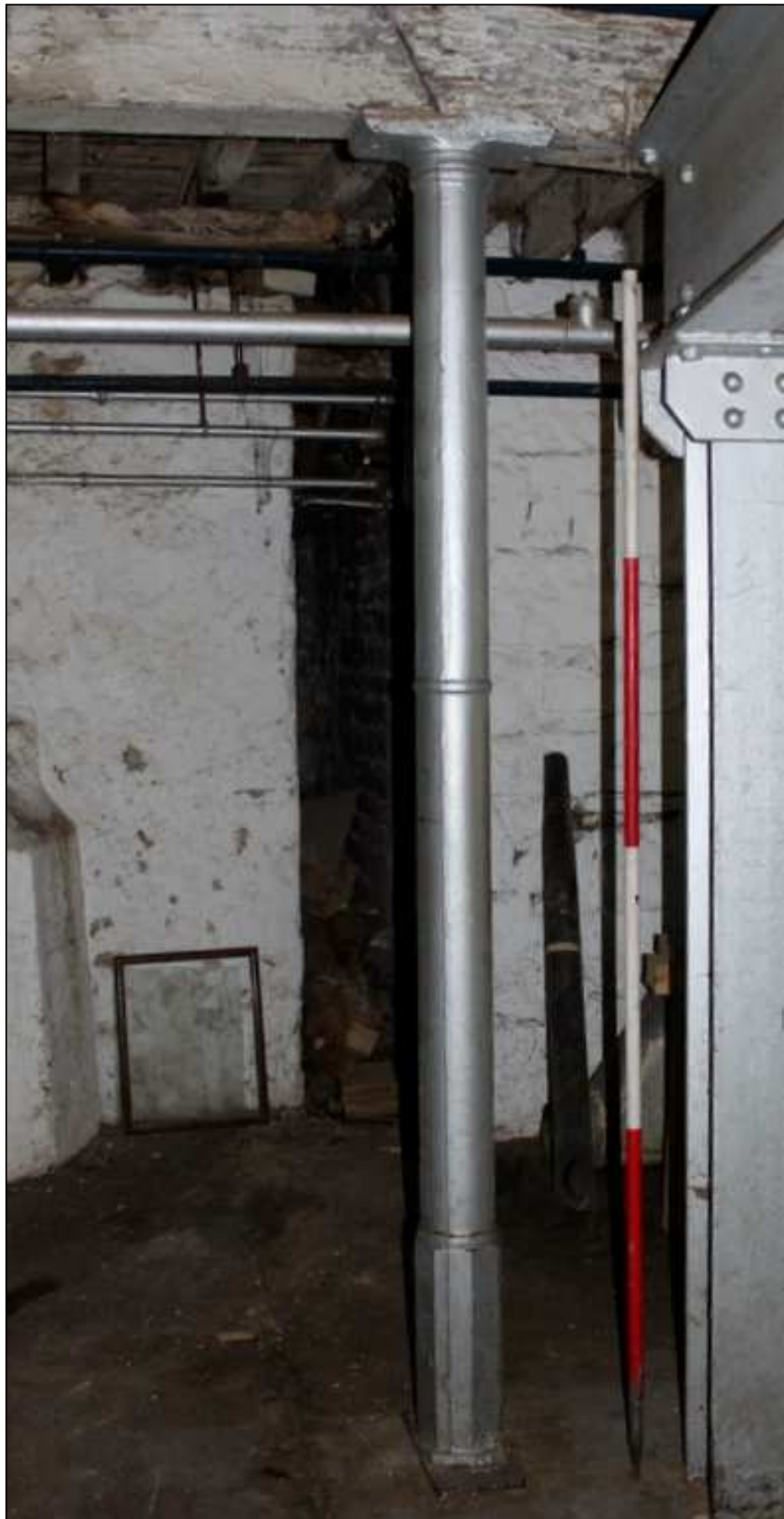
Plate 30: Column with astragal in shaft
