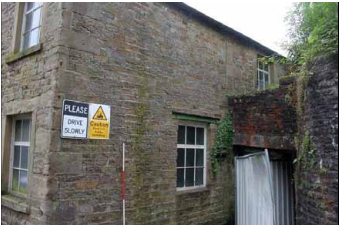
Plate 11: North wall of east wing and wall flanking headrace
