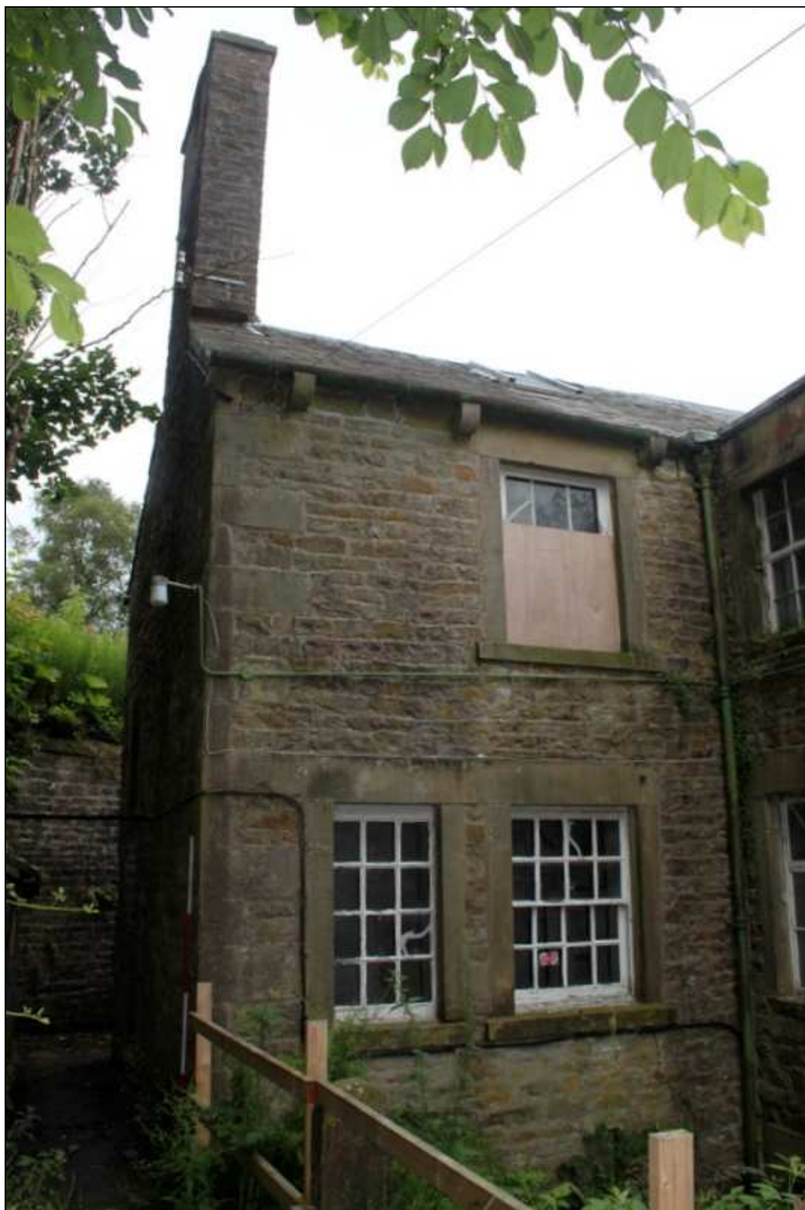
Plate 18: The west elevation of the tower, showing the 16-light window
