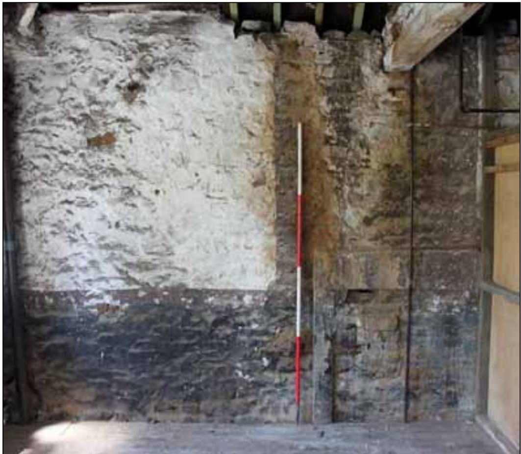
Plate 82: Jamb and lintel of fireplace in north wall of west wing
