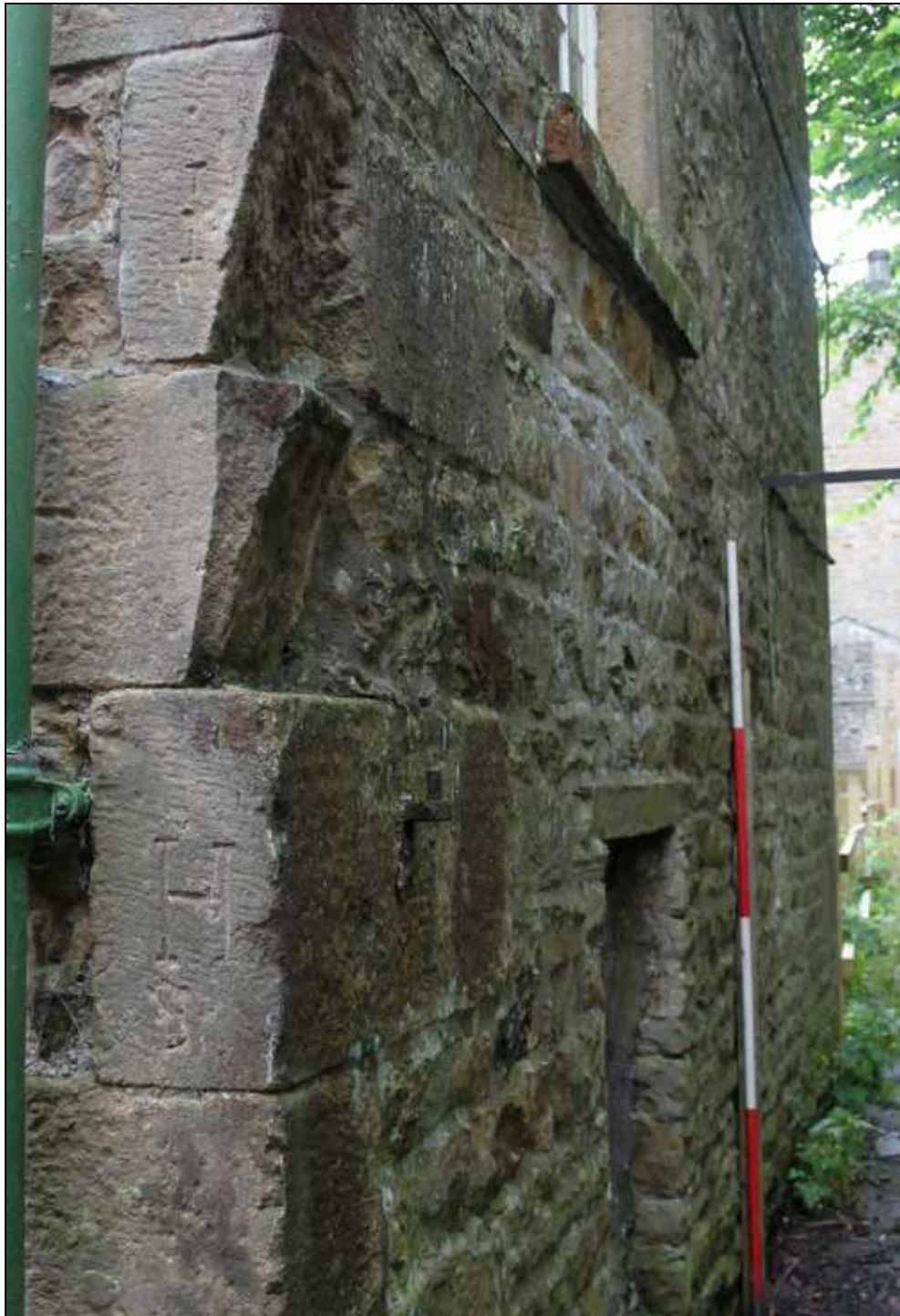
Plate 16: Mason's marks on stair tower quoins
