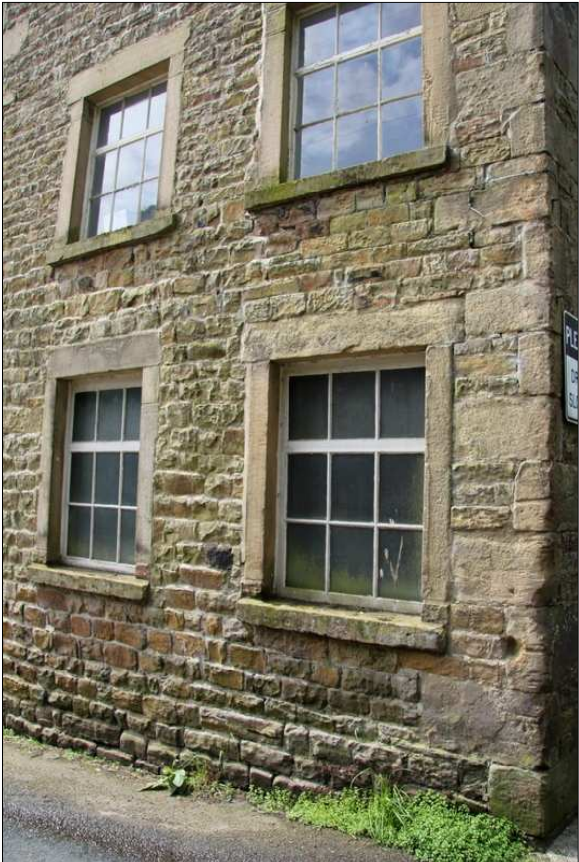
Plate 20: North return of the east wing, showing rebuilt wall and inserted windows
