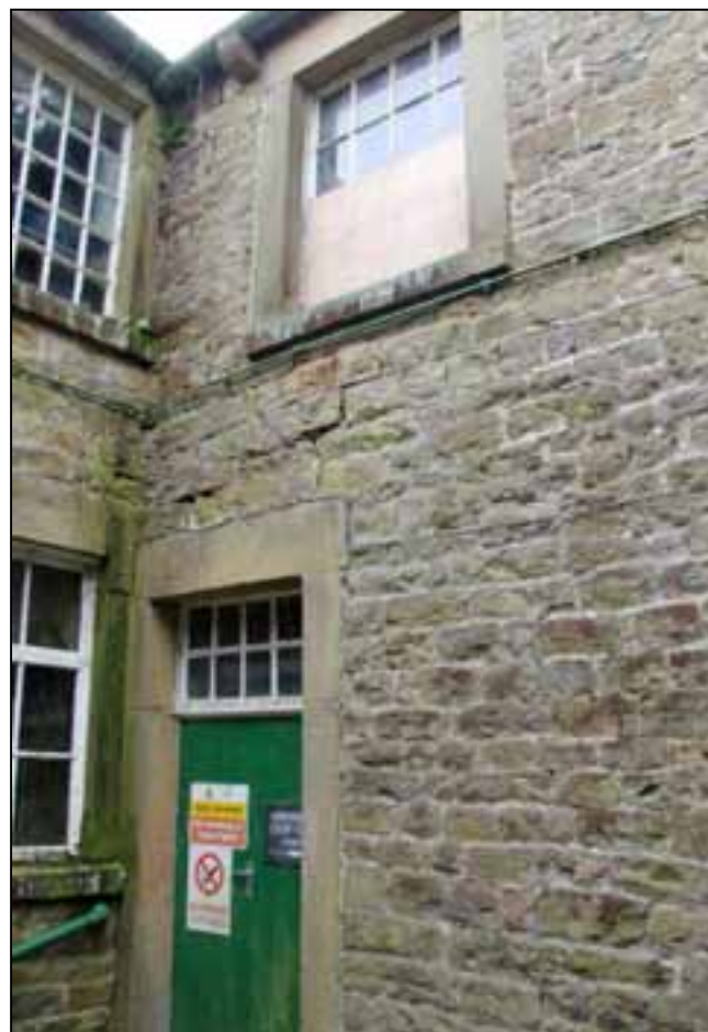
Plate 15: East wall of stair tower
