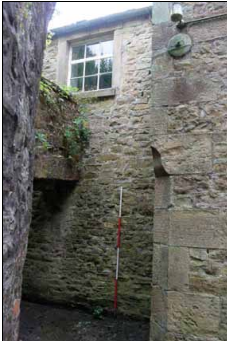
Plate 9: North wall of wheel house and chamfered return of main mill
