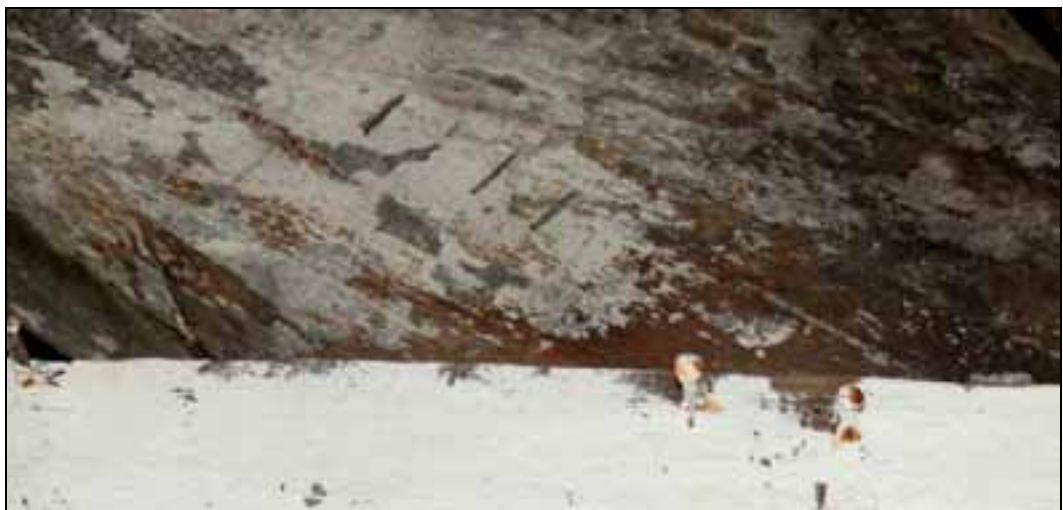
Plate 84: Chiselled carpenter's assembly marks
