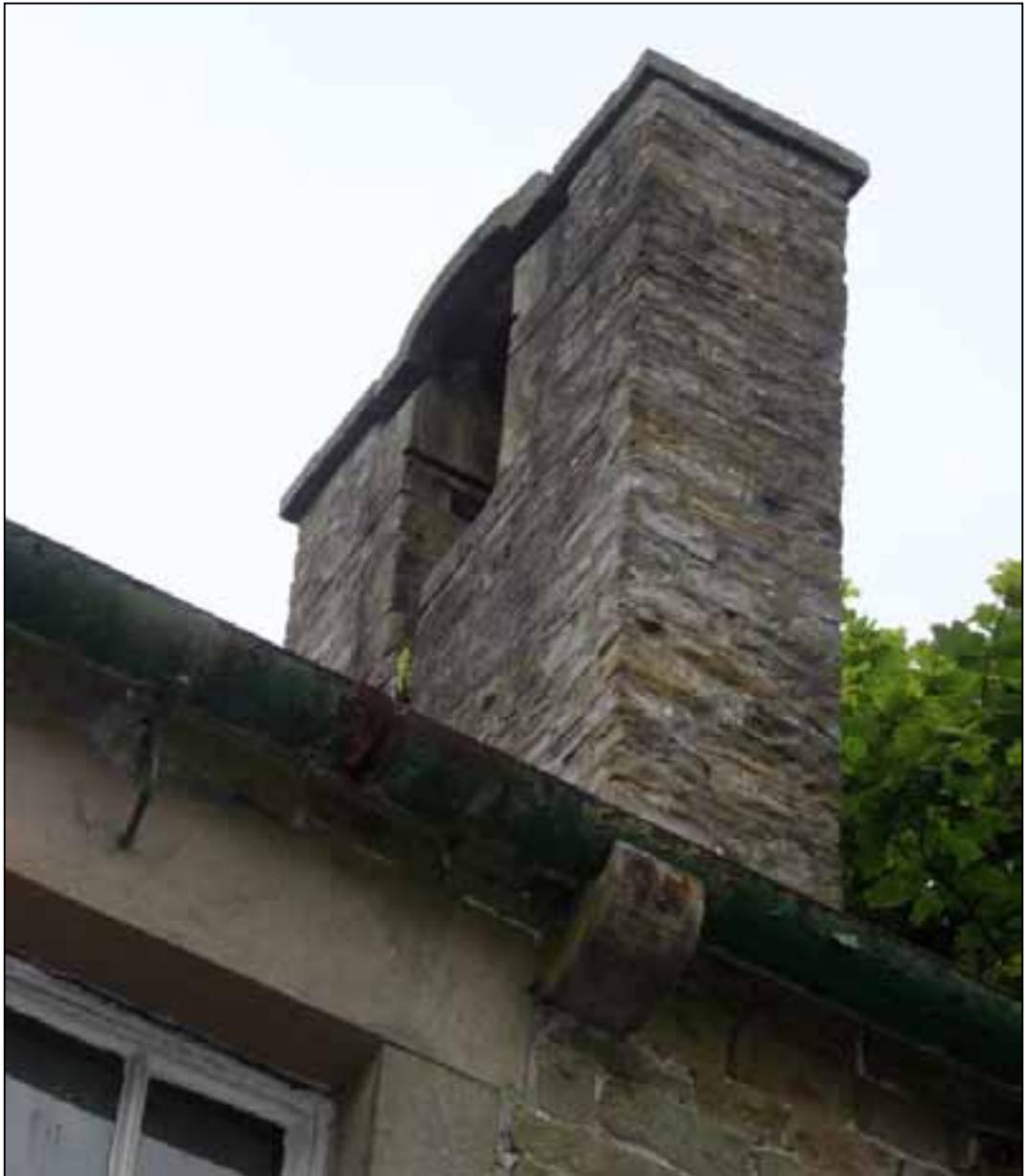
Plate 17: Bell cote above stair tower
