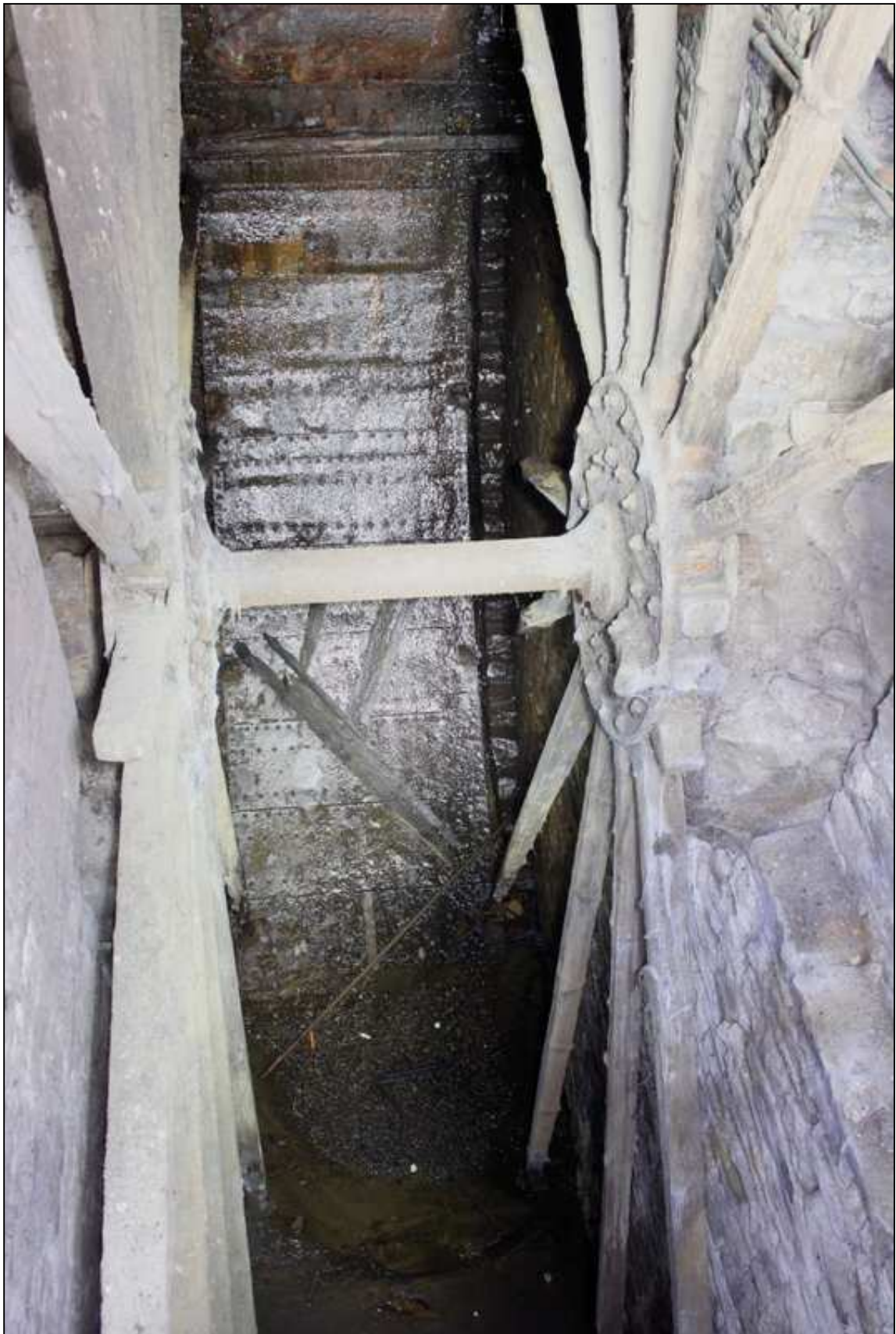
Plate 70: Axle and eastern bearing of waterwheel
