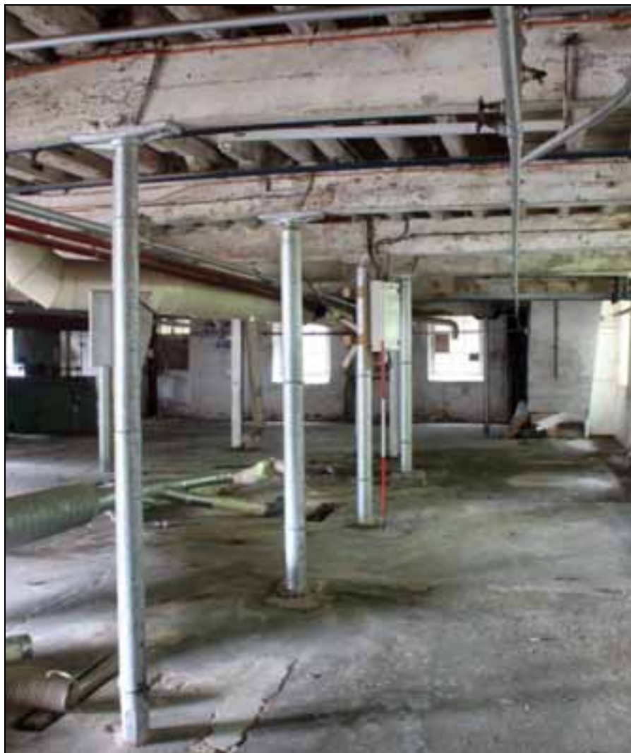
Plate 28: Inserted columns on the ground floor
