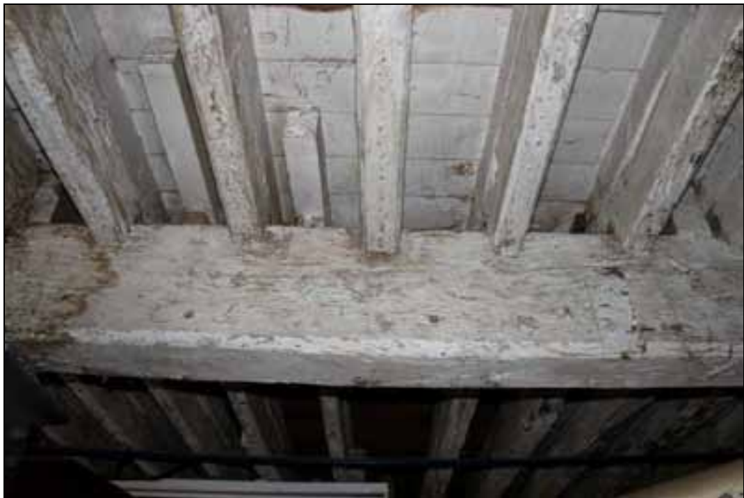
Plate 26: Large-scantling chamfered ceiling beams and exposed joists
