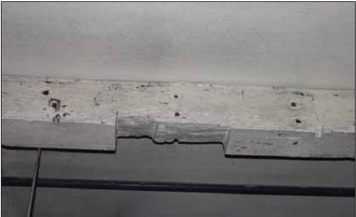
Plate 73: Evidence for original line shafting in east extension
