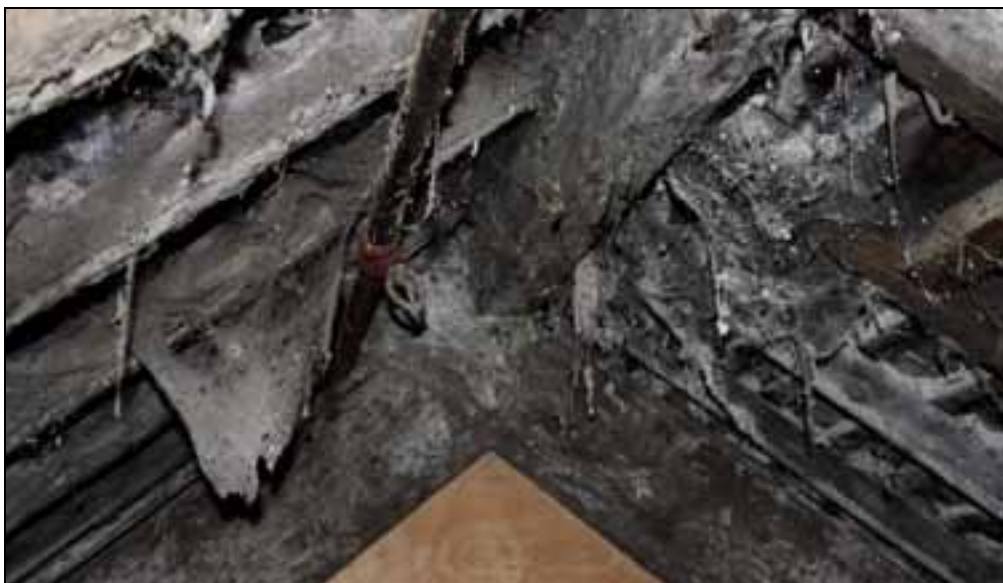
Plate 91: Apex of stair tower roof
