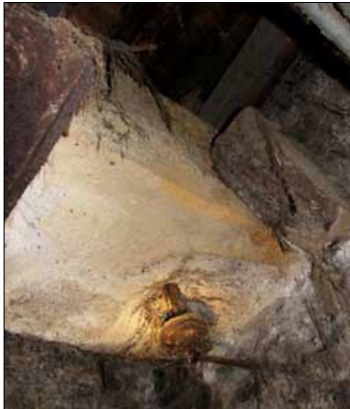
Plate 42: Large sandstone footstep for waterwheel gearing
