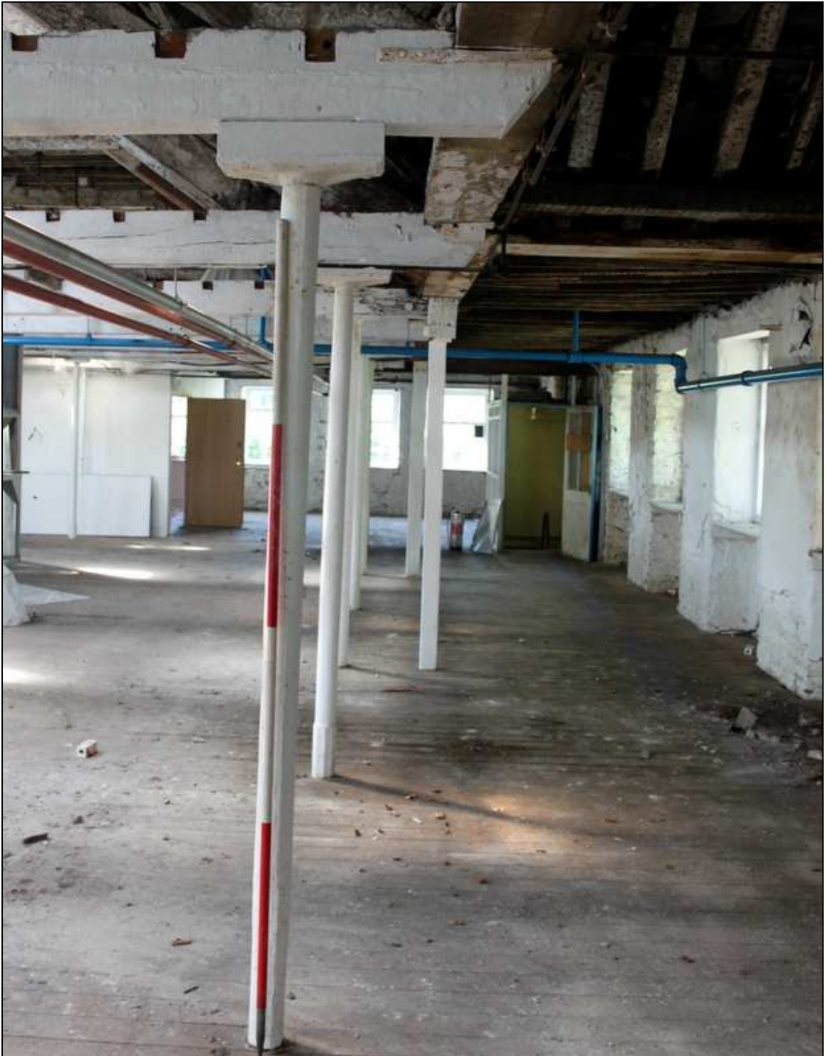
Plate 78: Second-floor columns supporting exposed beam ends
