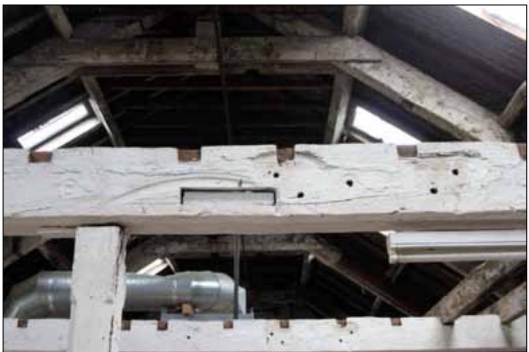
Plate 77: Drum scar and line shaft bolt holes, second floor
