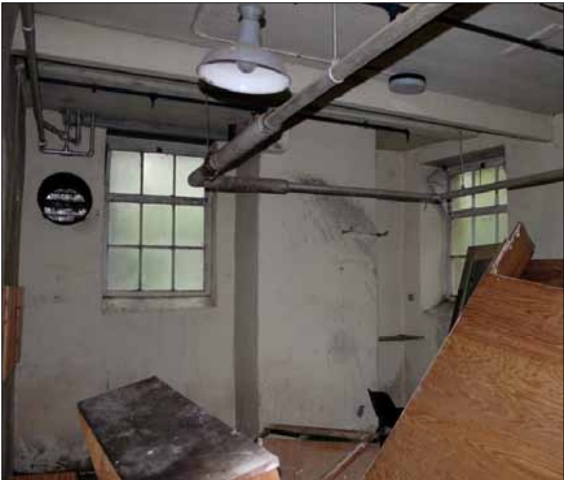
Plate 74: Chimney breast in repositioned north wall of east extension
