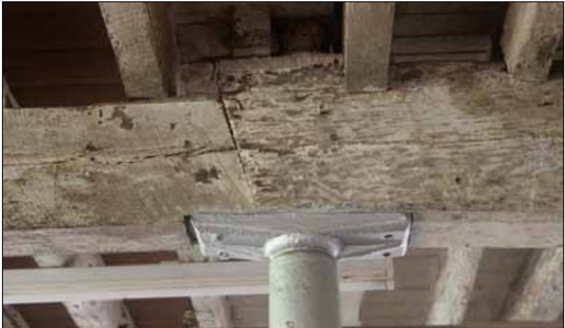
Plate 27: Simple scarf joint in ceiling beams above ribbed capital
