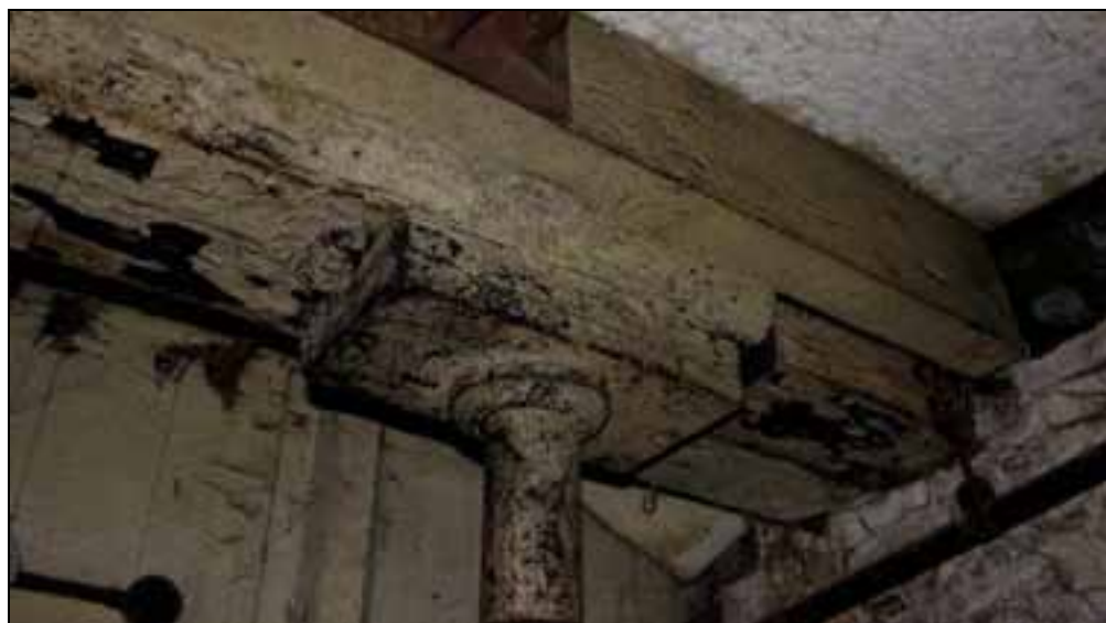
Plate 58: Column carrying scarf-jointed of extended ceiling beam
