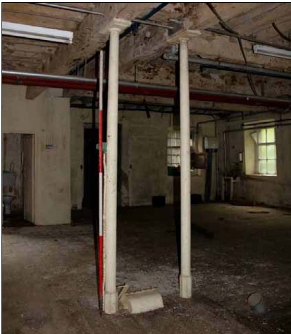
Plate 49: First-floor columns with octagonal-section feet
