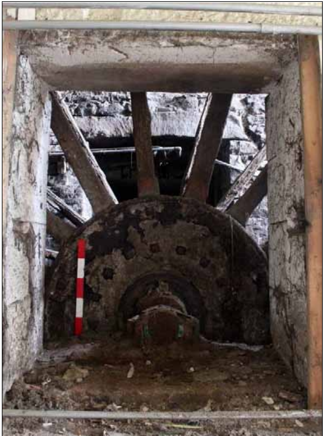
Plate 46: Waterwheel axle
