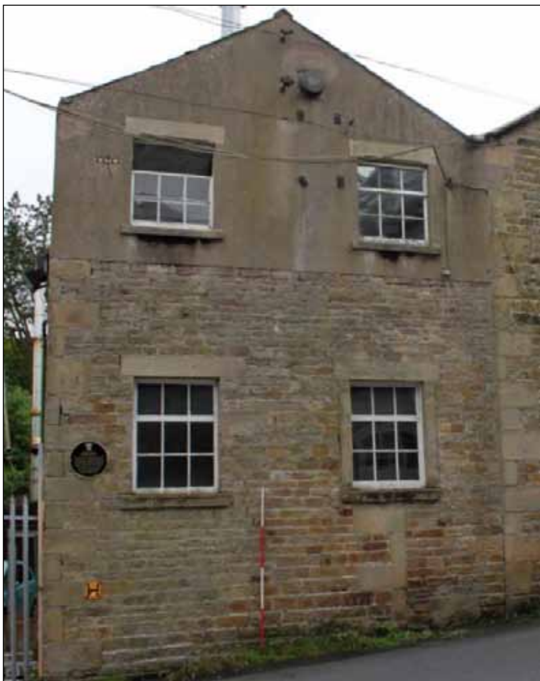
Plate 21: Southern extension to the east wing
