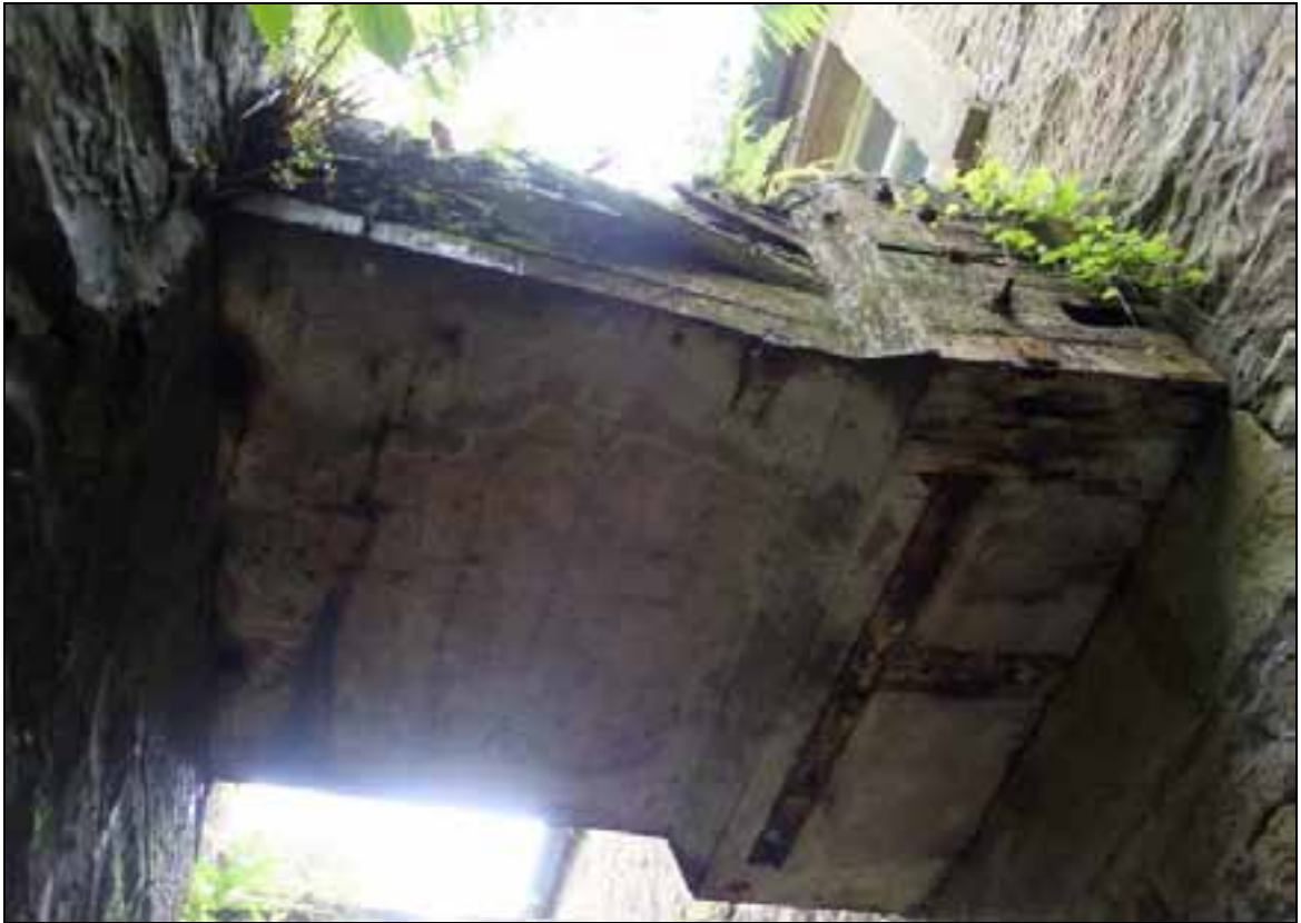
Plate 10: Concrete base of headrace
