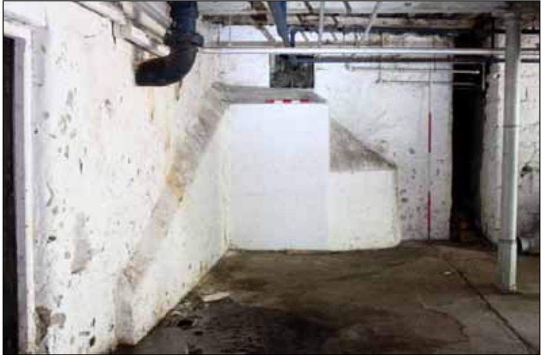
Plate 41: Substantial stone base for gearing footstep with line shaft end bearing box
