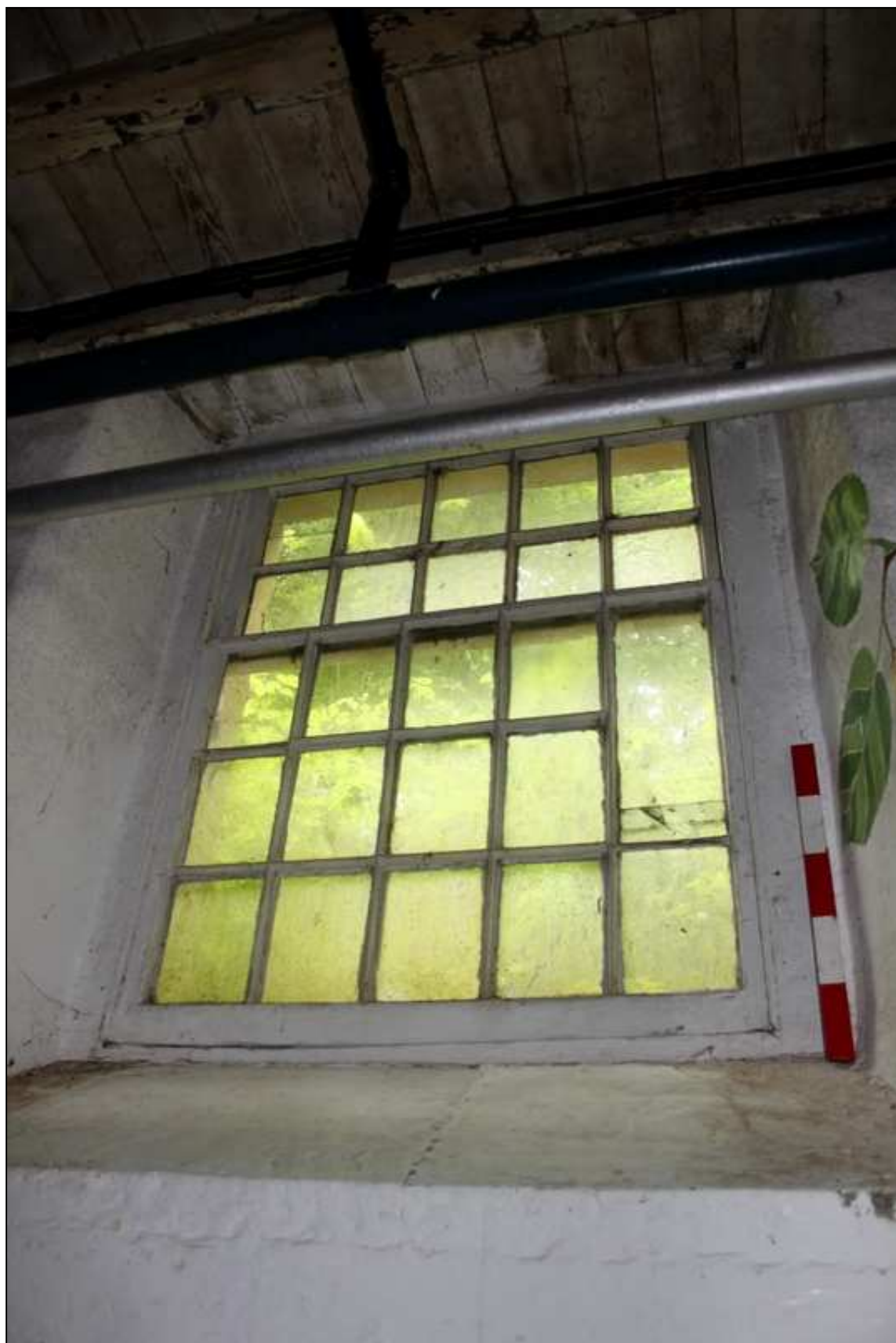
Plate 32: Vertical sash window in north wall
