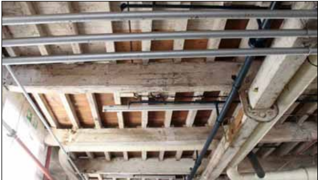
Plate 35: Additional longitudinal ceiling beam in west wing
