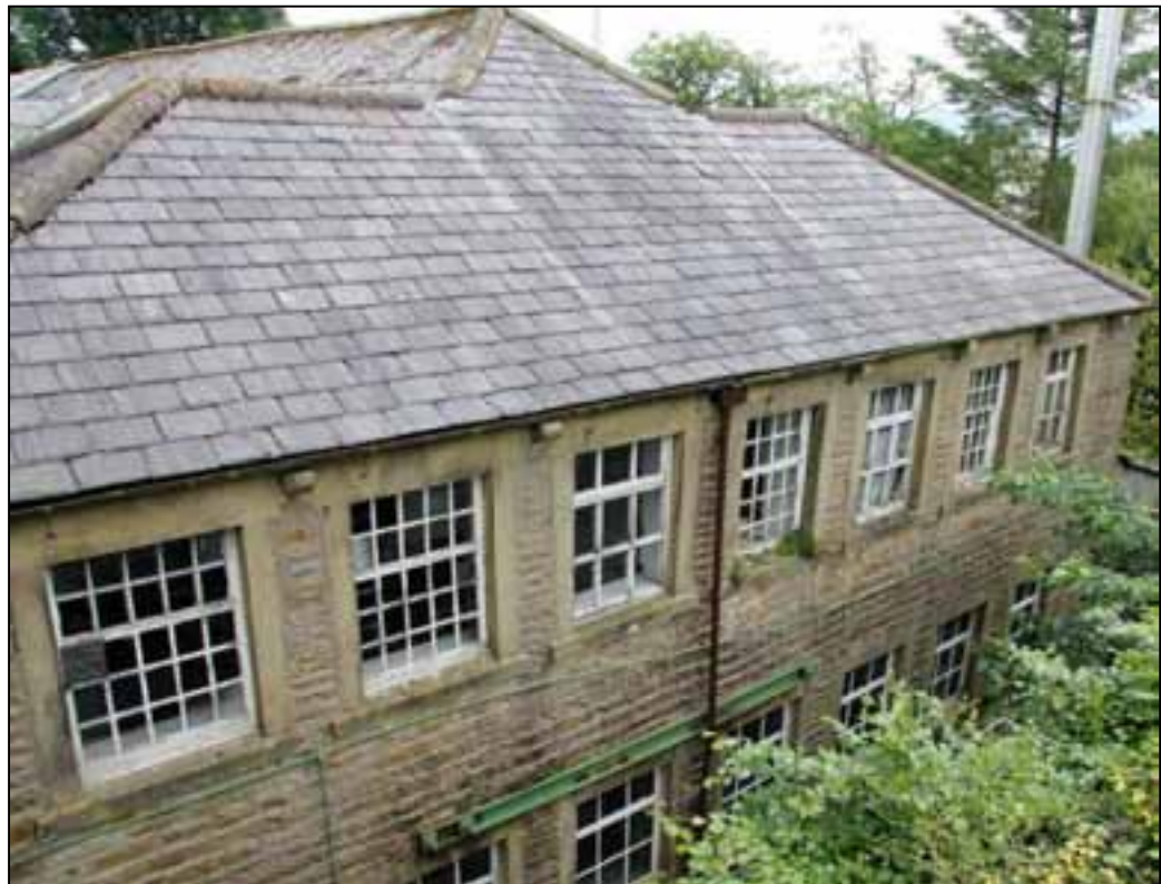
Plate 12: External west elevation of the west wing
