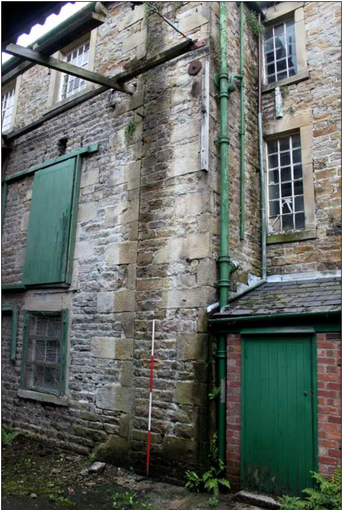
Plate 5: Quoined returns of west wing and privy tower
