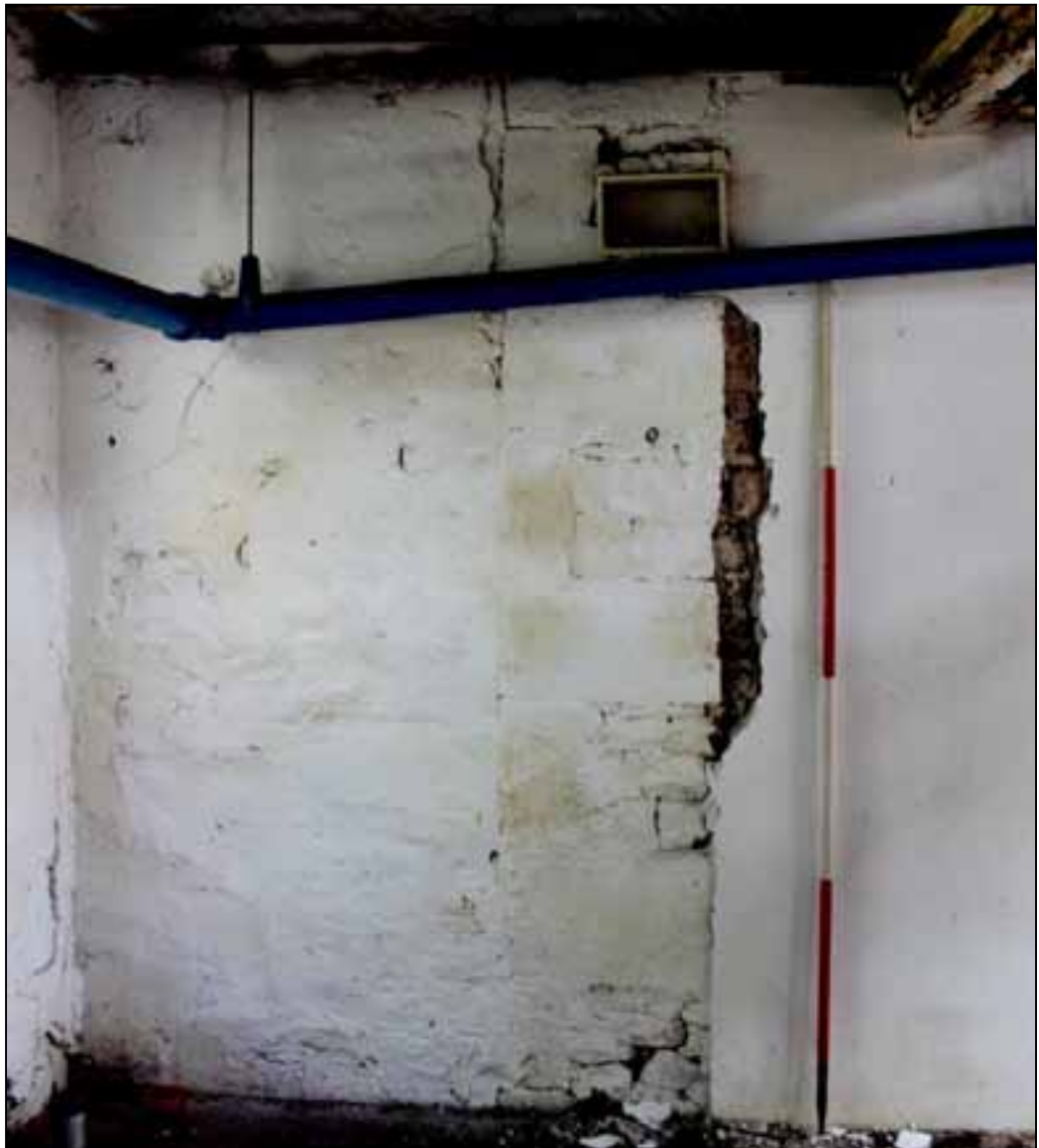
Plate 81: Quoins of wheel house in east wall of main mill
