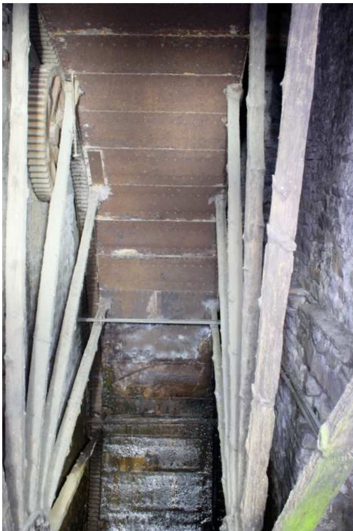
Plate 69: Extant waterwheel with slender timber spokes
