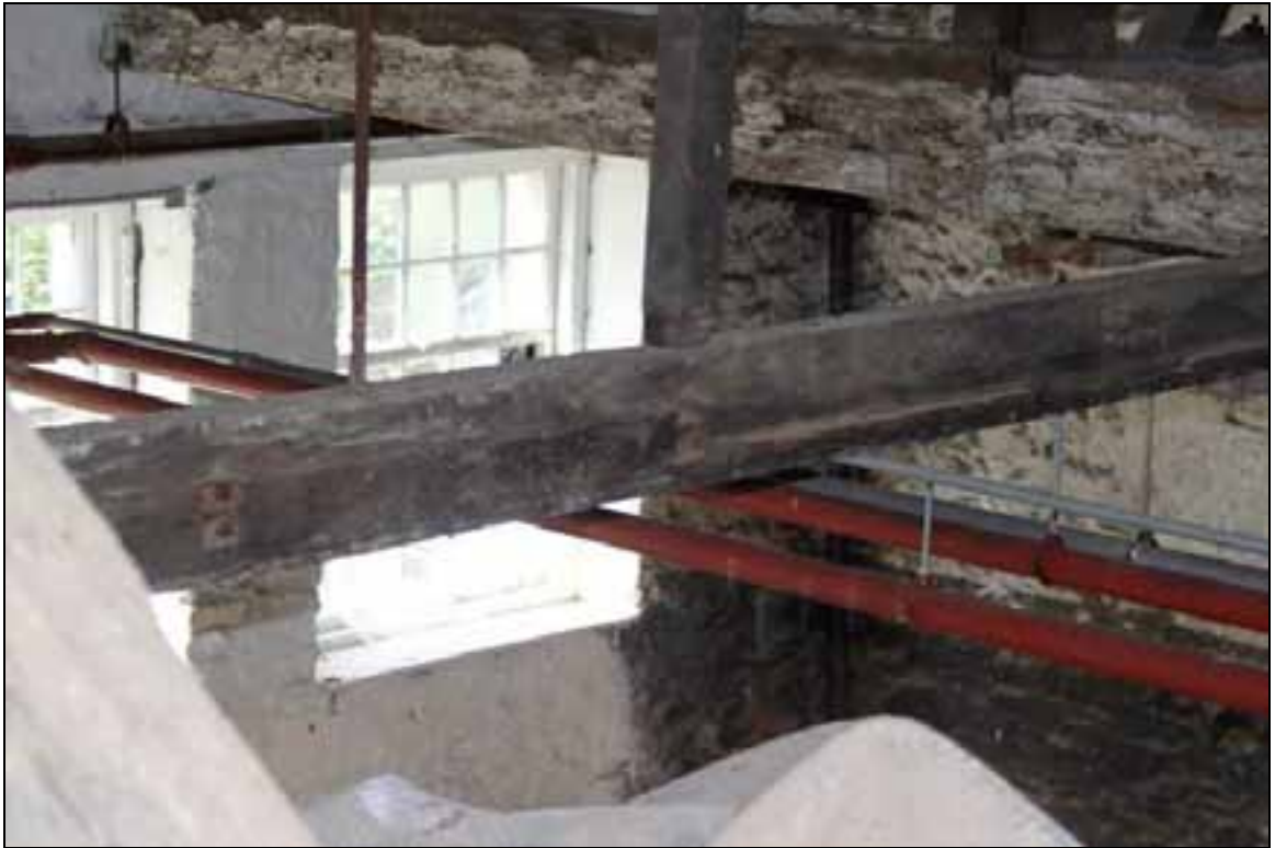
Plate 86: Mortices for ceiling joists above west wing
