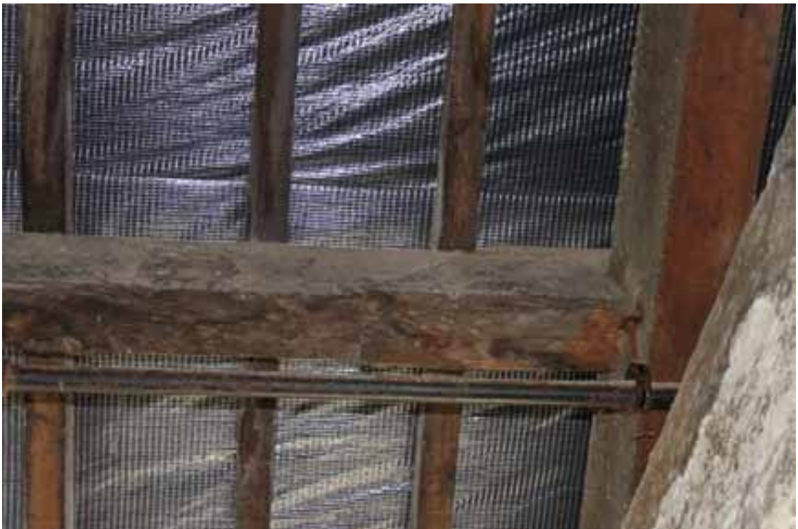
Plate 89: Scarf joint in purlin of west wing
