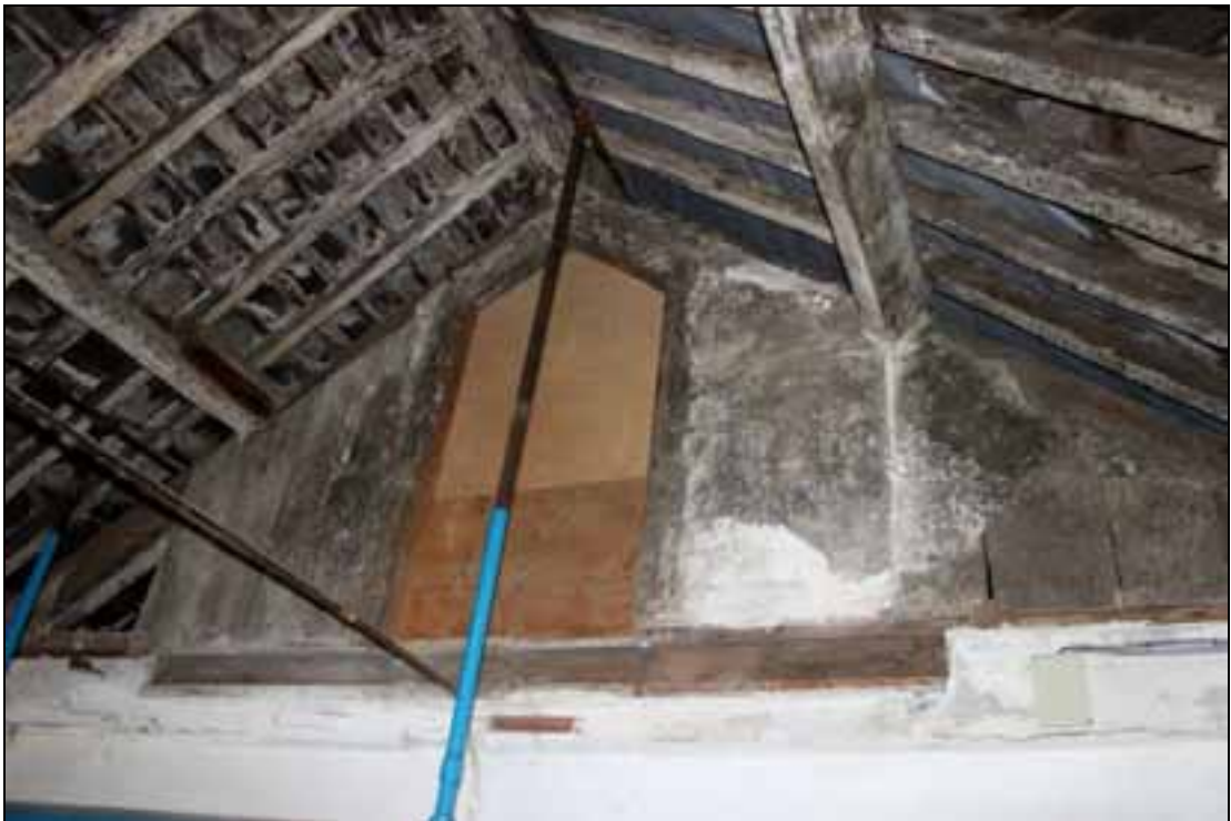
Plate 92: Doorway in attic above stair tower, with associated lath and plaster partitions
