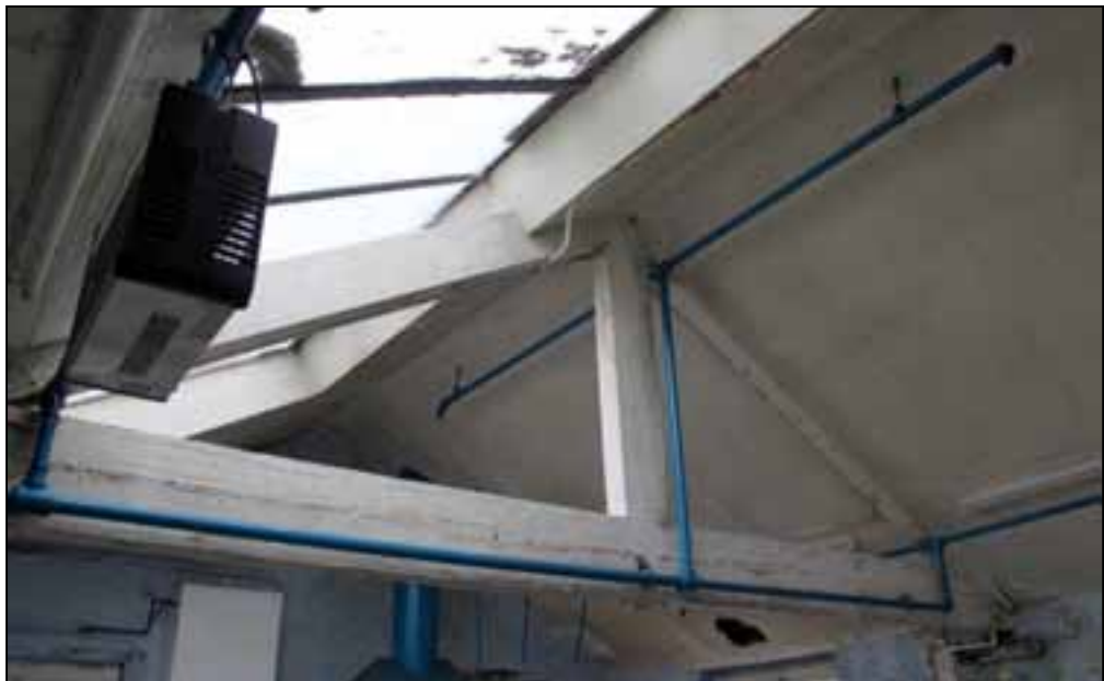
Plate 98: King post truss and glazing band above raised south extension
