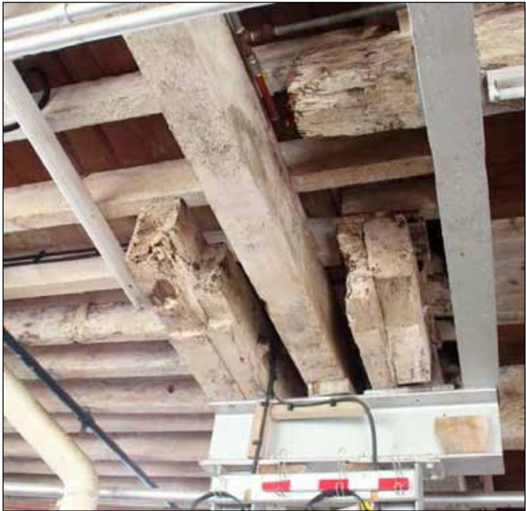
Plate 37: Close-set ceiling beams on late steel pad
