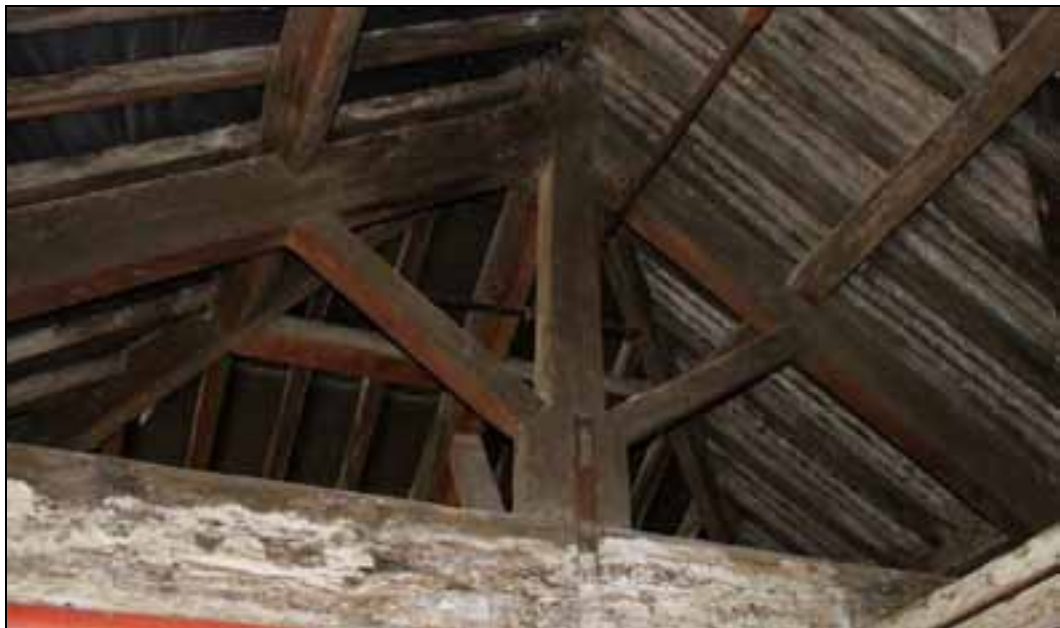
Plate 85: King post truss above west wing
