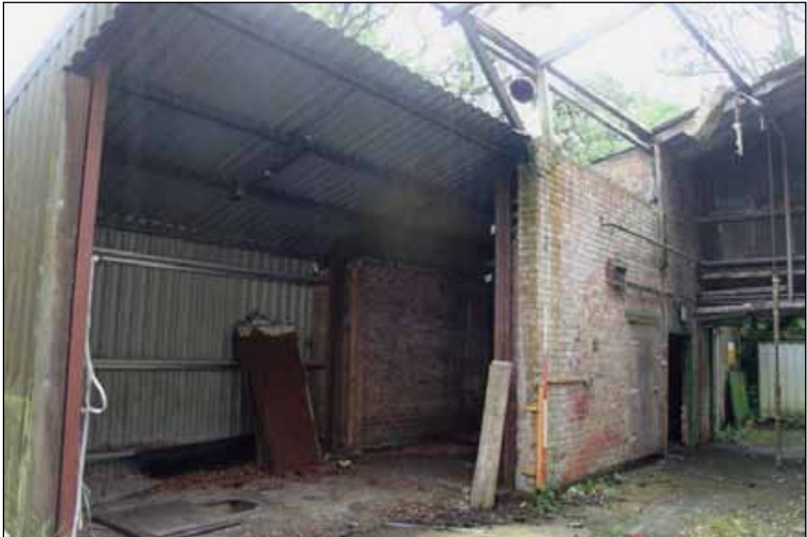
Plate 23: Remodelled store south of the west wing
