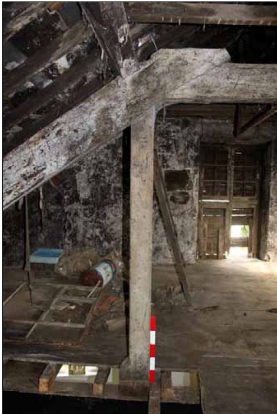
Plate 96: Queen strut truss above east extension
