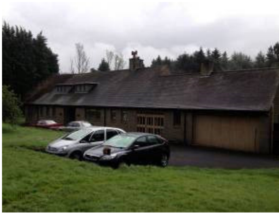
Existing Dormer Bungalow
