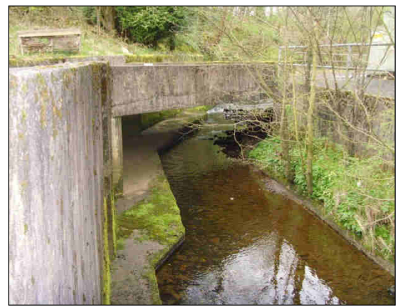
Site Bridge (1) – downstream face
