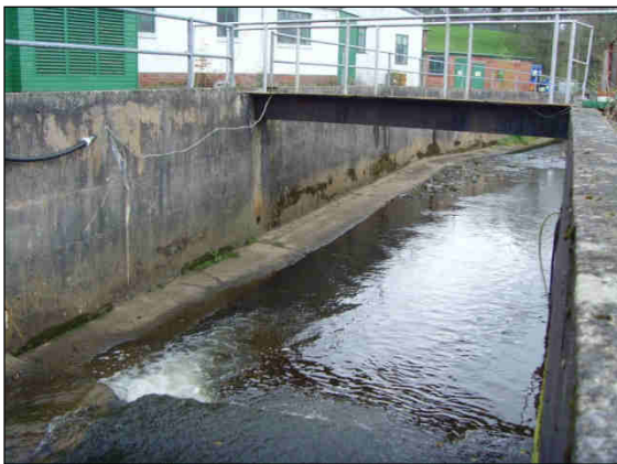
Site Bridge (2) – upstream face
