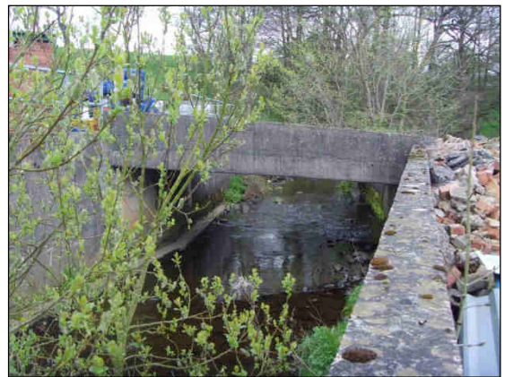
Site Bridge (3) – upstream face
