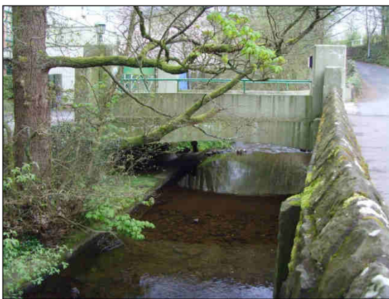
Main Access Bridge – upstream face
