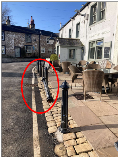
Figure 8 Damaged Bollard
