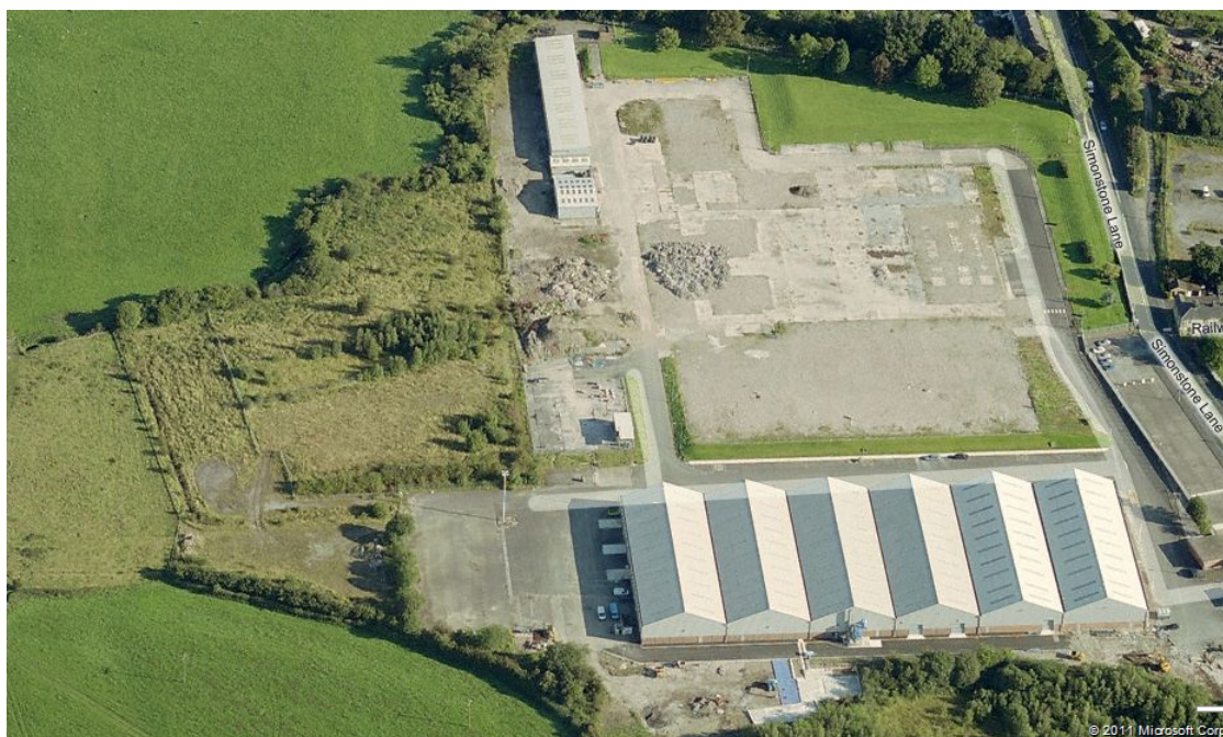
Fig 1: Site of former lagoons now made land to the west of the Mullard's works site. Note existing hedgerows to demarcate boundaries to the north-west and south-west
