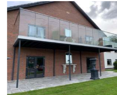
7. 1.8 metre High Glass Balustrade
