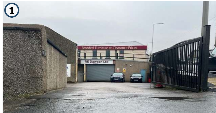
Image 1 - Access to lower level loading area from Pendle Road.
