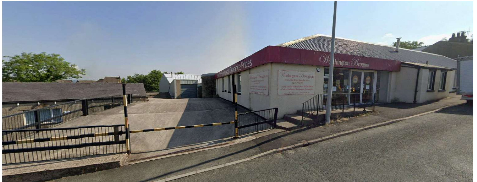
Approach Three - South west boundary showing existing building and loading bay area.
