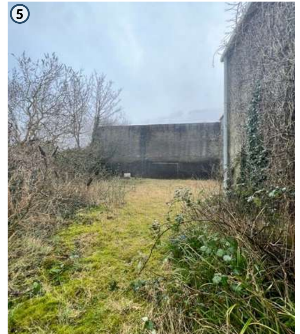
Image 5 - Courtyard on north boundary with grass and greenery.
