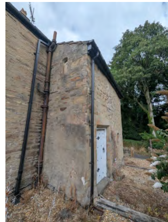
Figure 20 View of the projecting stair turret
