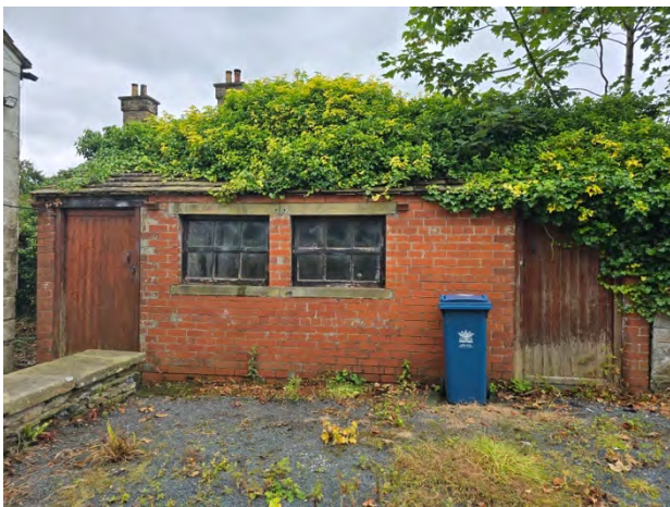
Figure 39: Exterior of the brick-built outbuilding
