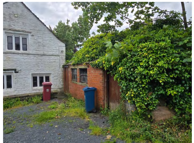
Figure 38: Exterior of the brick-built outbuilding
