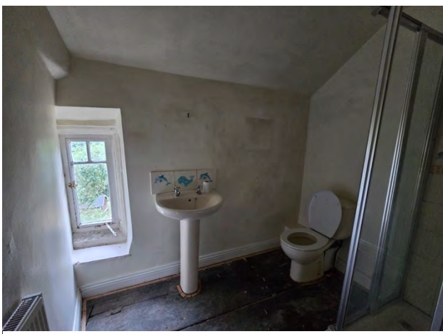
Figure 14: Example first floor bathroom
