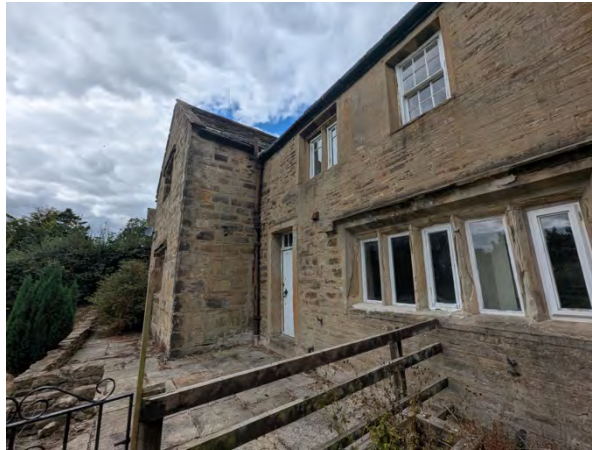
Figure 21 View of the now shared window
