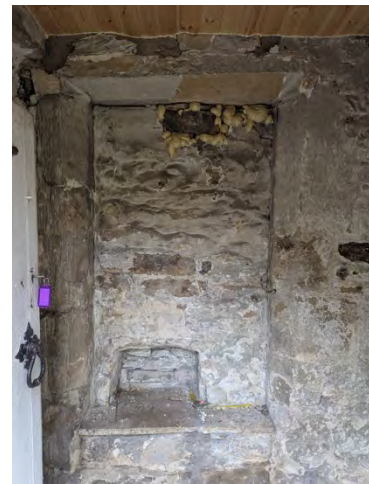
Figure 37 Internal shot of the stair turret
