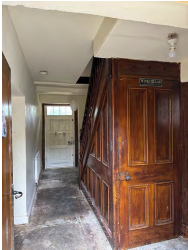
Figure 6: View of the ground floor through passage
