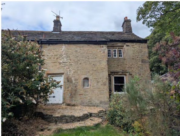
Figure 19 View of the principal elevation
