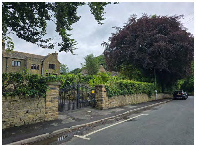
Figure 41: View of the west facing elevation of the study site from School Lane
