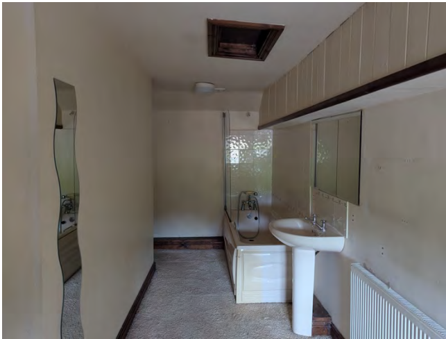
Figure 34 View of the bathroom
