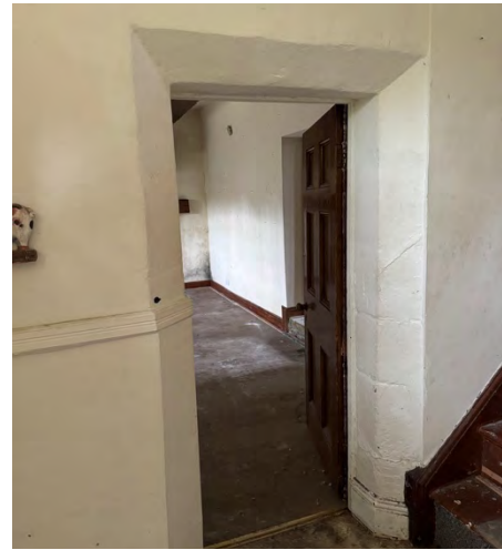
Figure 10: View of the chamfered internal doorways on the ground floor
