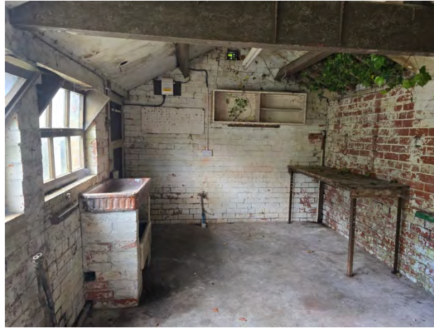
Figure 40: Interior of the brick-built outbuilding
