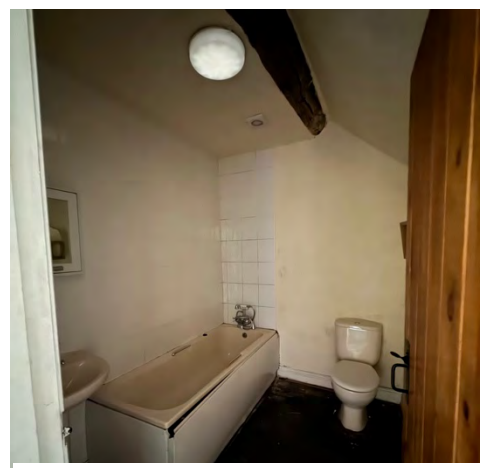
Figure 13: Example first floor bathroom
