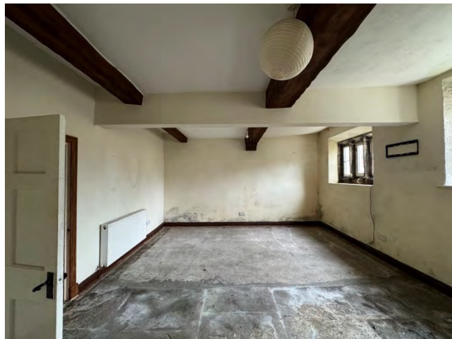
Figure 5: View of the rear sitting room
