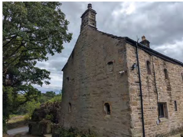
Figure 18 View of the east facing elevation
