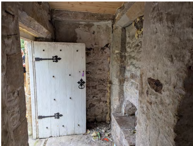
Figure 36 Internal shot of the stair turret
