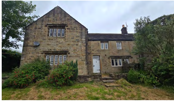
Figure 2: Principal south facing elevation of Cockshutts Farmhouse
