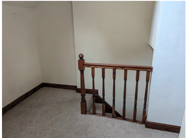
Figure 29 View of the staircase and landing
