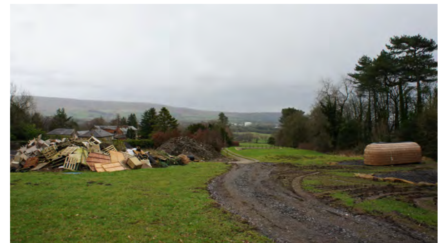
SPI View from the site, looking south towards Eaves Hall and Pendle Hill in the distance
