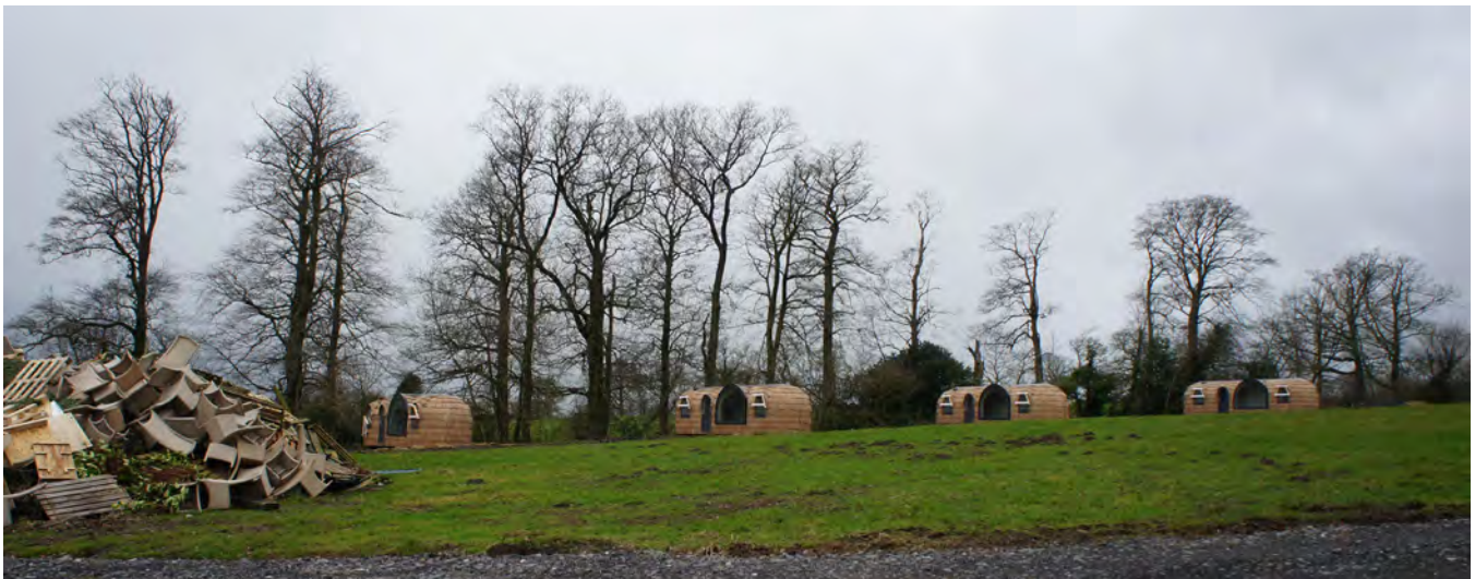
View from the centre of the development site looking west, showing the already installed eco-lodges
