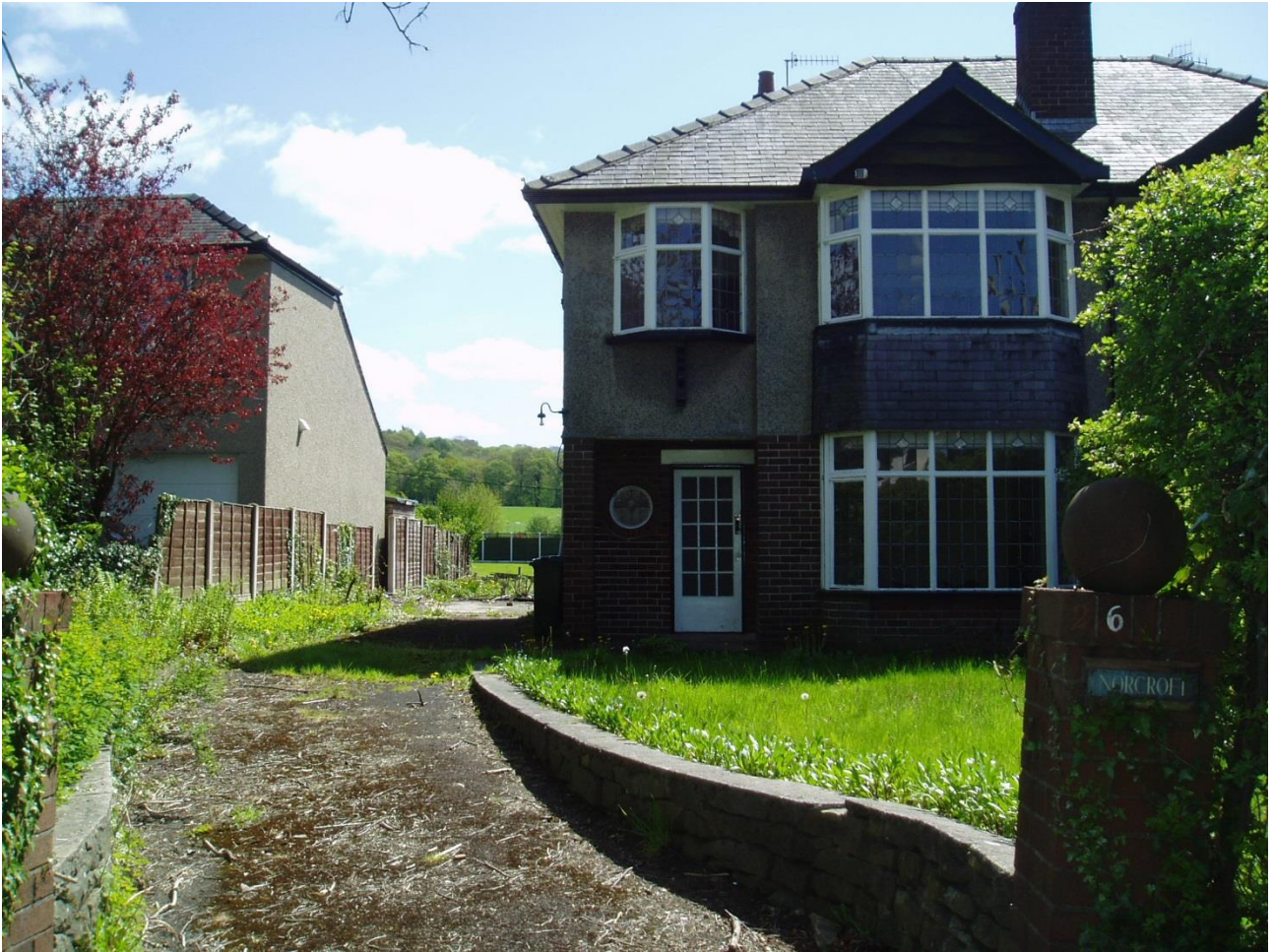
8 Front elevation of 26 Clitheroe Road and blank gable to the extension at 28 Clitheroe Road.
