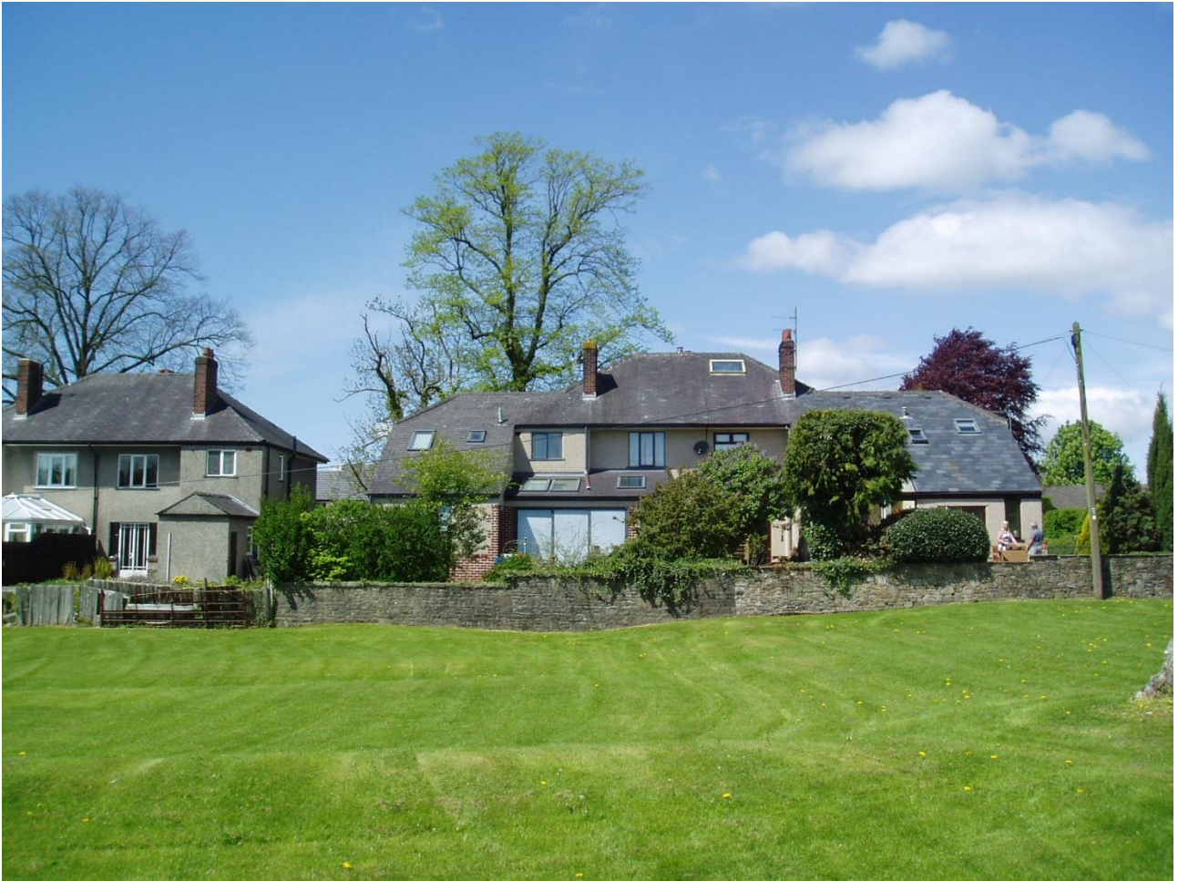
2. Large rear two storey and single storey extensions at 28 and 30 Clitheroe Road
