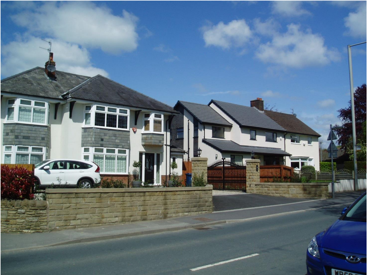
4. 19 Clitheroe Road ridge not set down and extension set back slightly
