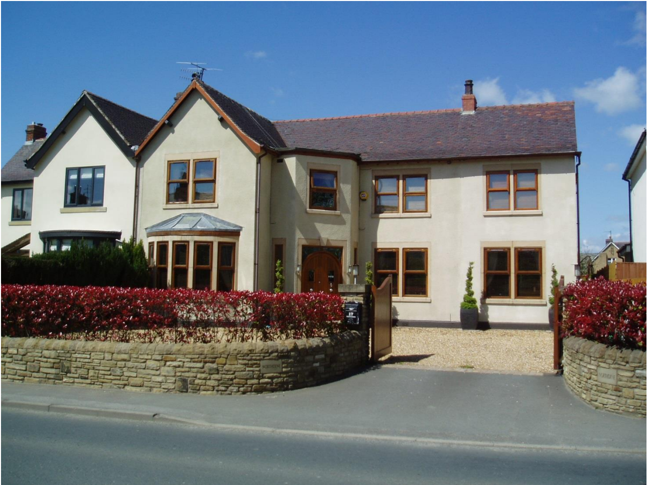
5. 17 Clitheroe Road two storey side extension ridge not set down and elevation not set back.
