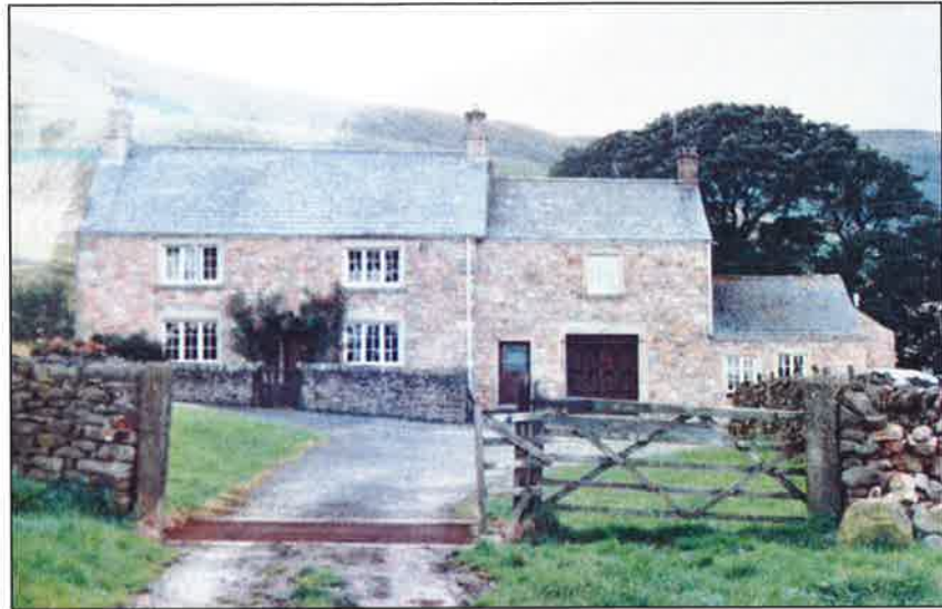
Photo 2: Photograph of 1980s/1990s, showing garage occupying north-east end
