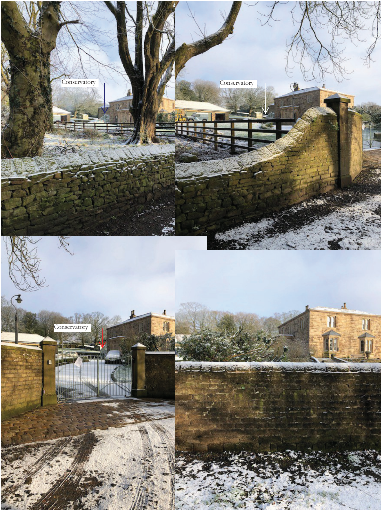
Site viewed from south along thoroughfare.
