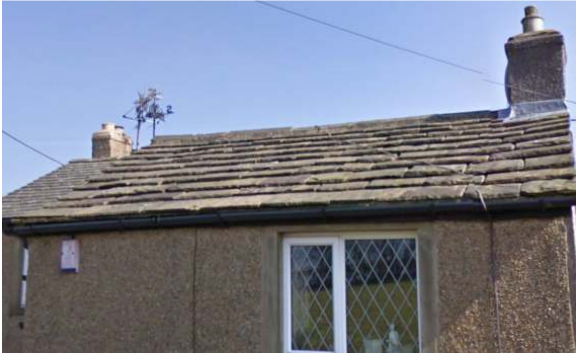
Photo 3: Photo of surrounding roofing materials
