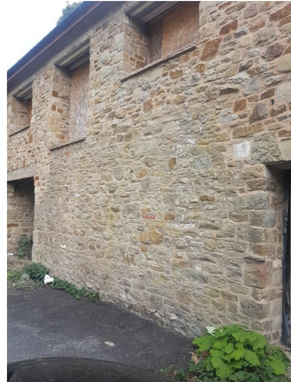
Image 4 – the rear of the site, showing irregularities in the stone and mortar
