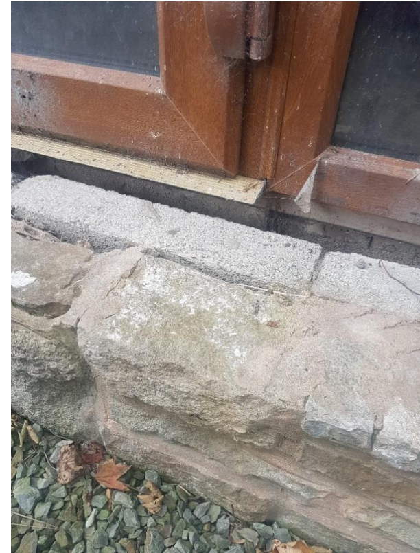
Image 11 – Evidence of the building being reskinned, as there is a new layer of concrete blocks behind the existing stone. The bottom layer of stone has new mortar, which is differing in colour to the old.
