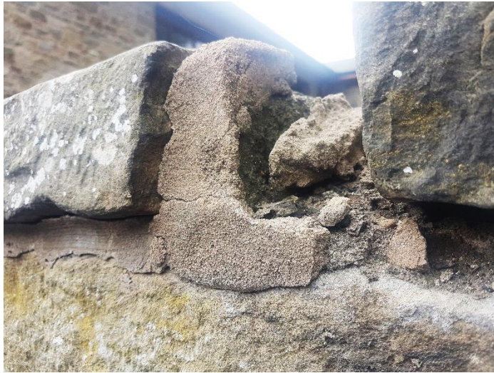
Image 10 – close inspection of courtyard wall showed new mortar applied on top of old and much of it had evidently been re-built
