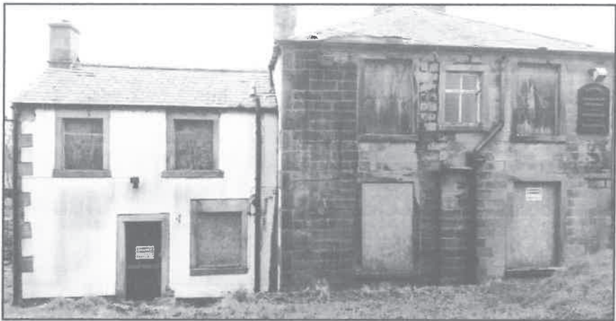
Figure 7) Later C19th eastern addition with rear service outrigger. The combination of main front part and rear outrigger indicates that this was probably a separate dwelling.
