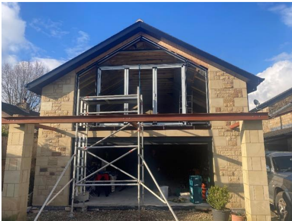
Photograph 2.3: south elevation of appeal development as constructed. The piers and steel work to the front, designed to support a terrace, are proposed to be removed
