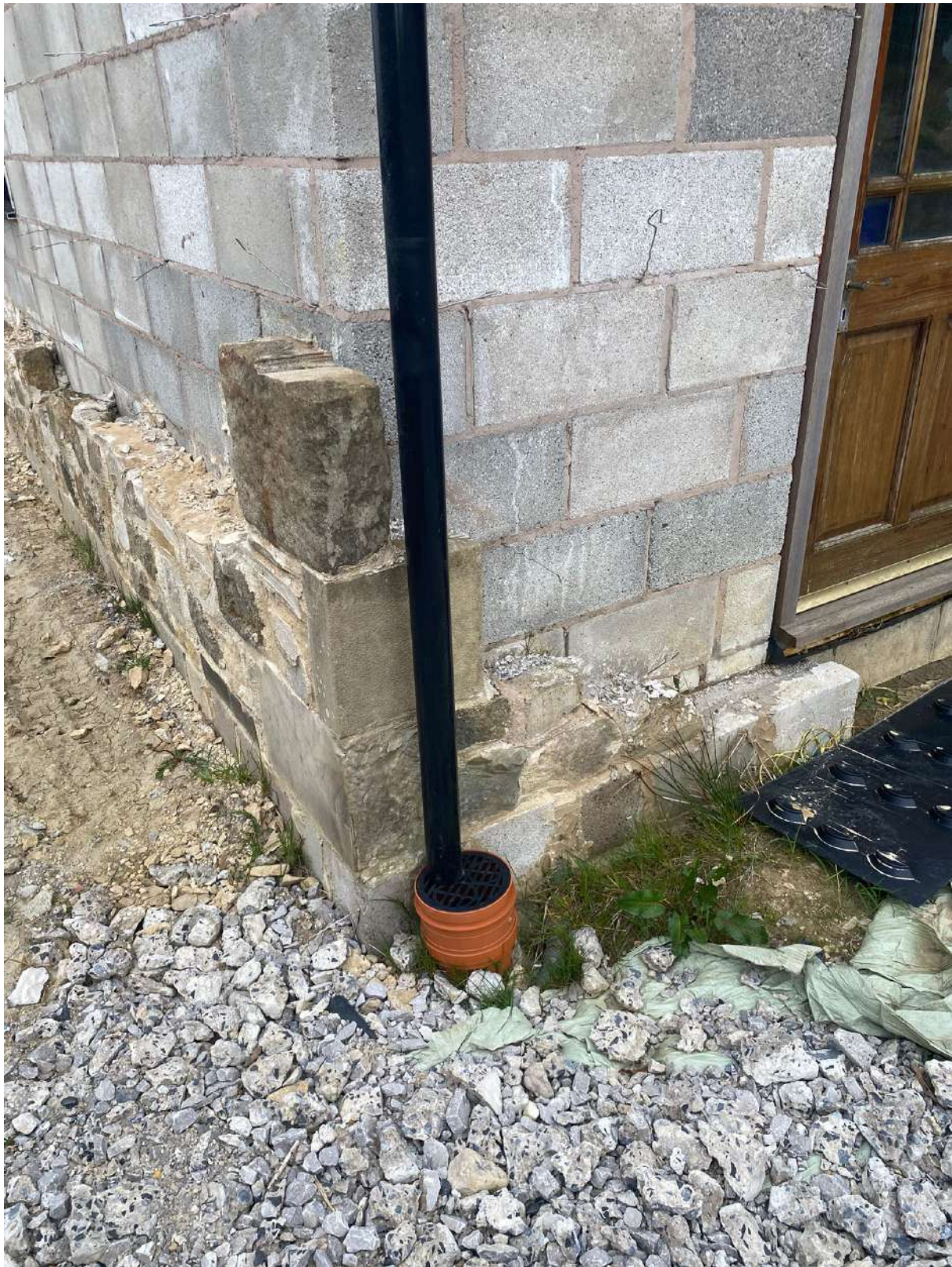
Drainage as installed
