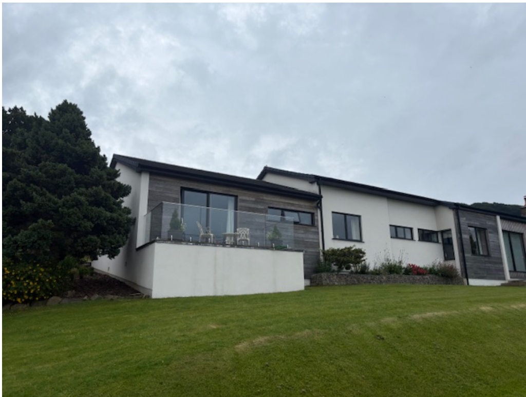
No 34 – Render, Zinc cladding, aluminium windows, corten steel door
