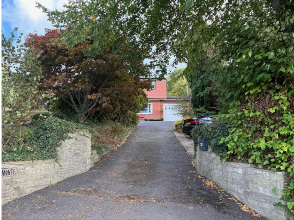
No 44 – Red tiled cladding, brickwork
