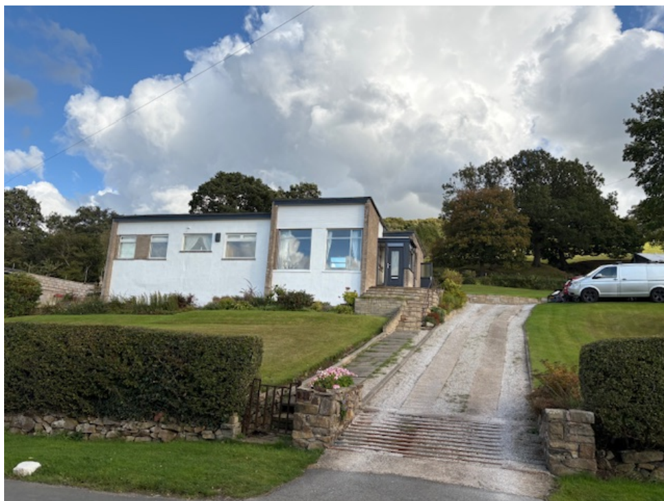
No 38 – Render, brickwork
