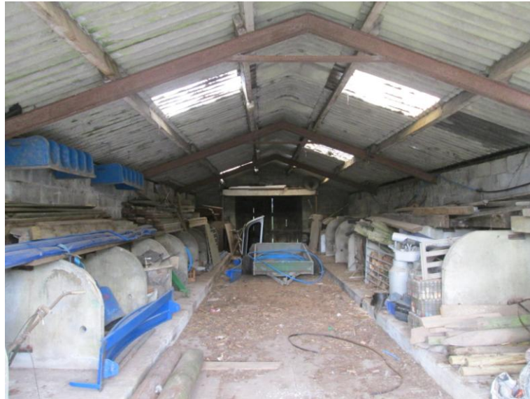
Photo 3 – Building A – Internal View
