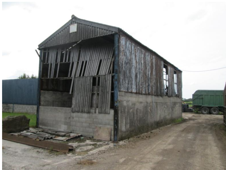
Photo 4 – Building B, from South East
