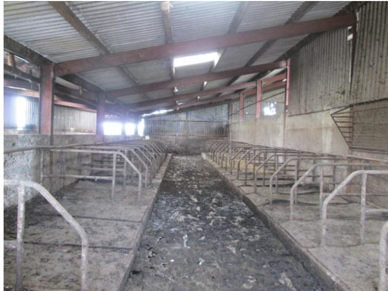
Photo 11 – Building C – Span 2
