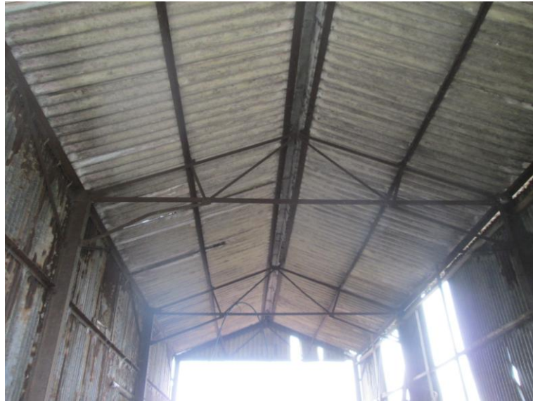
Photo 5 – Building B – Roof Structure
