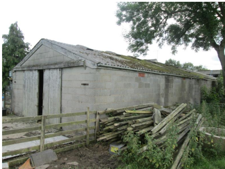
Photo 2 – Building A, from North West
