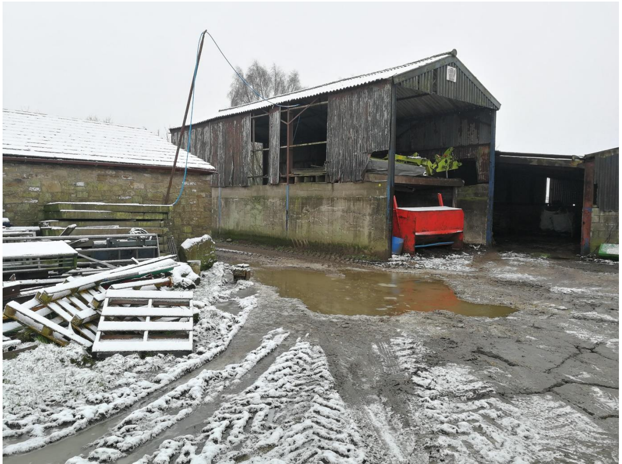
Image 6: View towards storage shed and neighbouring outbuilding
