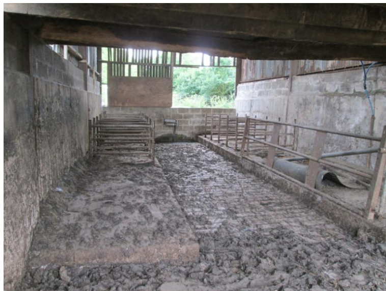
Photo 6 – Building B – Floor
