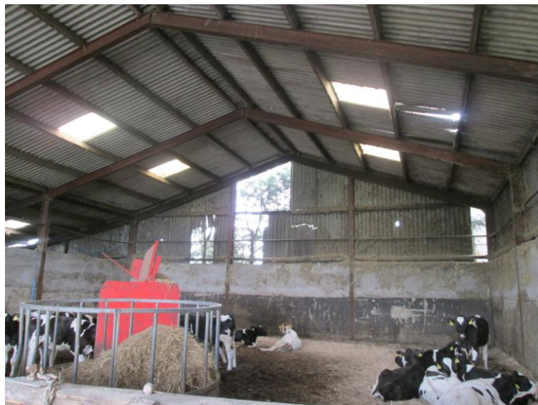
Photo 10 – Building C – Span 1
