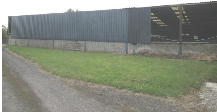
Photo 9 – Building C – South East Wall
