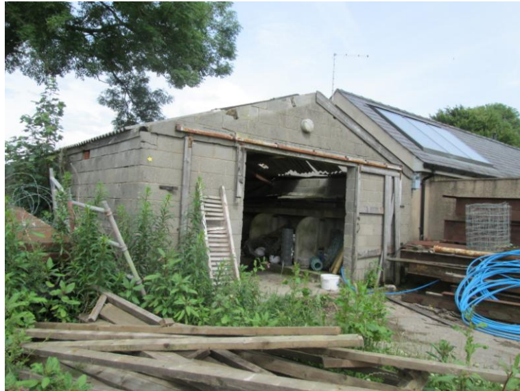
Photo 1 – Building A, from South West
