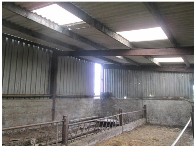
Photo 12 – Building C – Span 3
