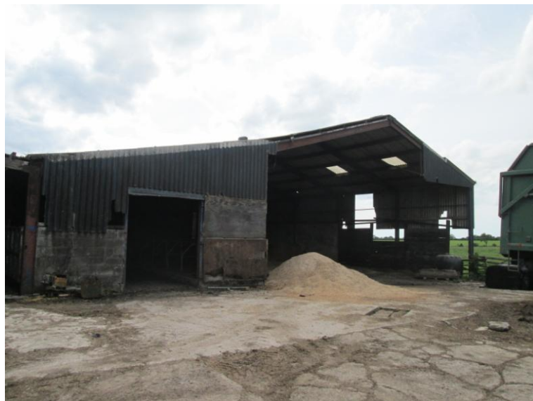
Photo 8 – Building C – North East Wall
