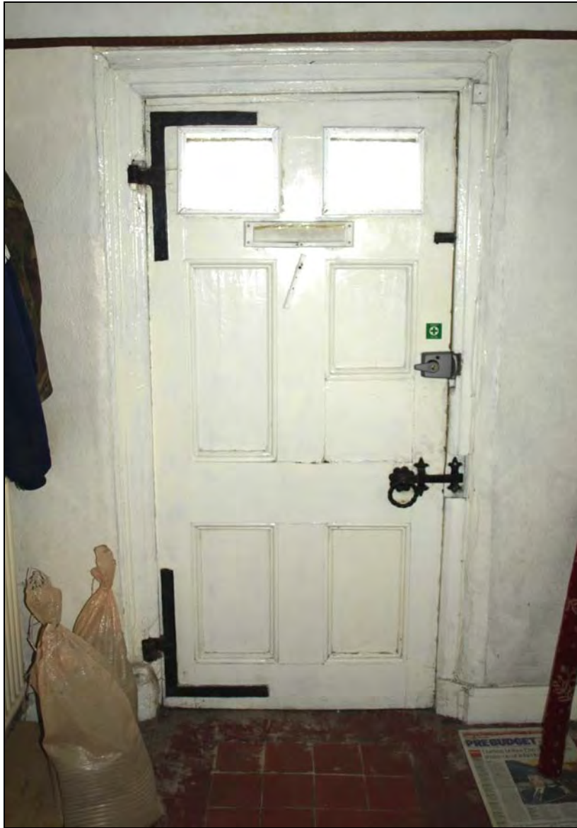
Photo 3: Rear of front door: note L-hinges
