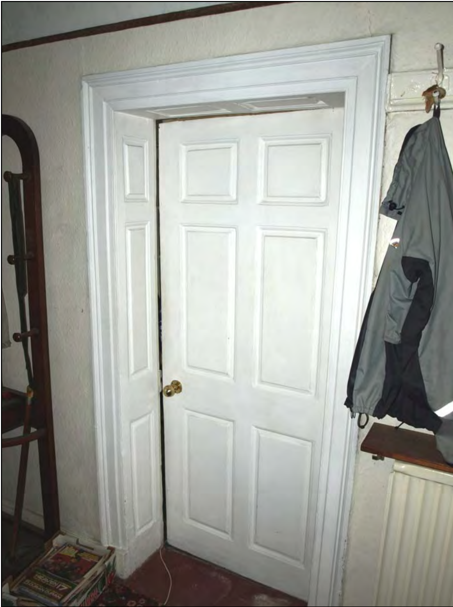
Photo 5: Typical six panel door and architrave, raised and fielded panels
