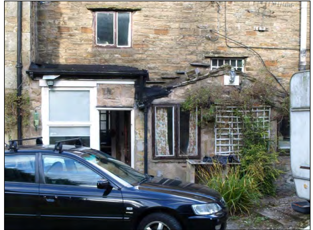
Photo 10: Back kitchen at foot of rear elevation: 19th century part under stone slate roof to right, 1980s addition under flat roof at left
