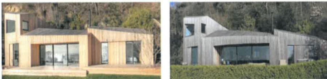
Figure 2: Images showing difference in appearance following the accelerated weathering using SiOO:X Wood Protection
