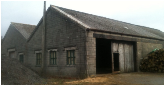
North and South west elevation, main entrance door.
