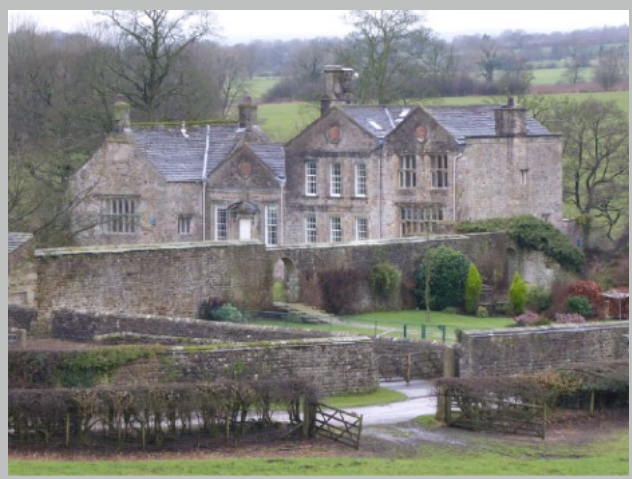
Plate 27. Bashall Hall with its walls
