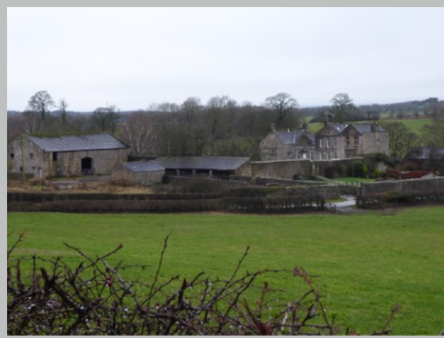
Plate 26. Bashall Hall with ensemble of farm buildings in front
