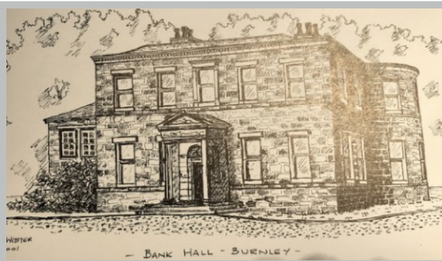
Plate 13. Bank Hall, Burnley - Rebuilt 18th C
