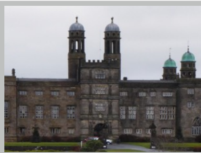
Plate 37. Four tiers of pilasters on frontage of Stonyhurst
