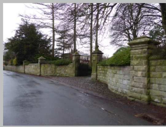
Plate 19. Entrance walls and cusp-topped piers with rusticated bases to Glebe House, Slaidburn
