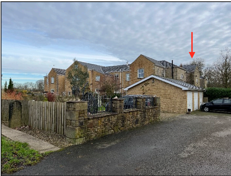
Figure 13: Woodfold Park Farm, seen from the south-west. The original elevation can be seen on the right (arrow), the projecting bays of the rest of the building, to its left in this view, are modern additions and sit outside the historic footprint of the building. The more complicated elevation on this side is alien to the original restrained architecture and has undermined the historic integrity and legibility.
