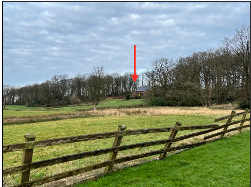
Figure 7 (right): The walled kitchen garden with its pair of modern houses, seen from just south-west of the mansion. Here it is clear how much taller than the walls the houses are. They may have been designed to look like functional bothies and backsides, but their scale makes that a nonsense – and ensures they are prominent in the landscape.
