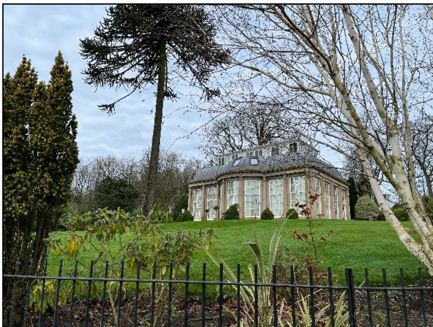
Figure 9: A closer view of the orangery with its incongruous modern roofline.
