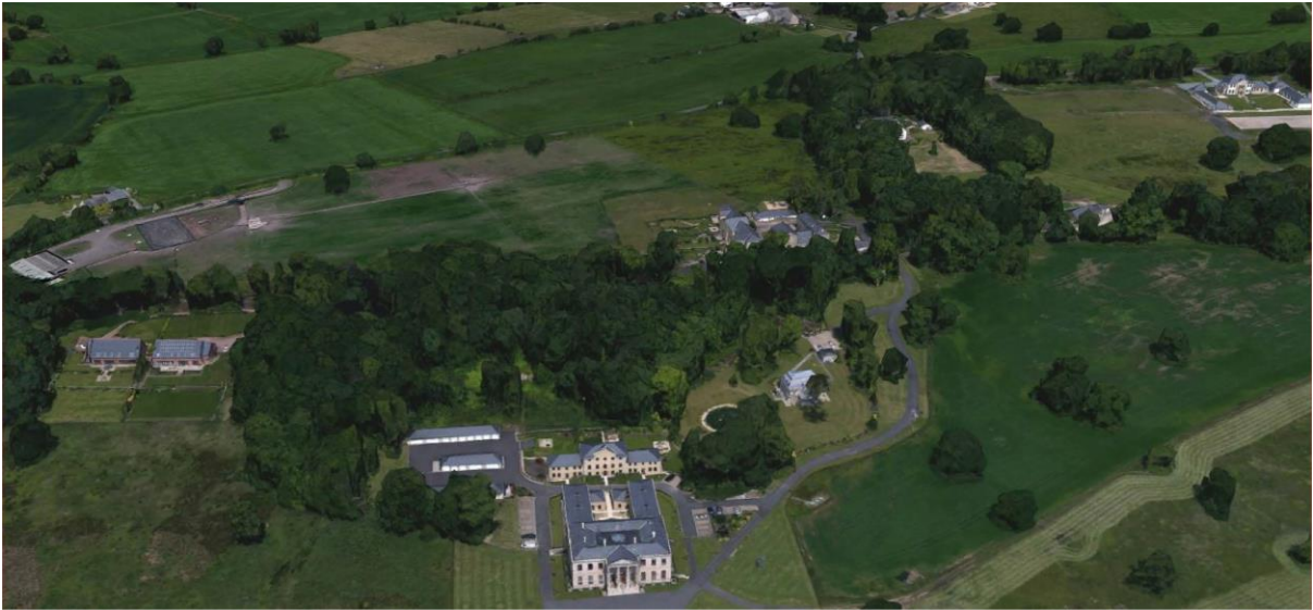
Existing aerial view from the south
