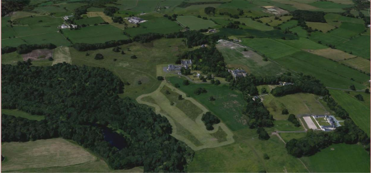
Existing aerial view from the east
